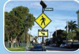
Rapid flashing beacons
