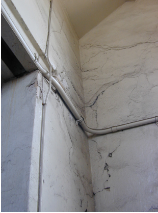
Figure 23: Damaged and settling plaster interior walls of the 1900 Pumping Station. The abandoned electrical conduit has been removed by the HAF in association with Louis Vuitton.
