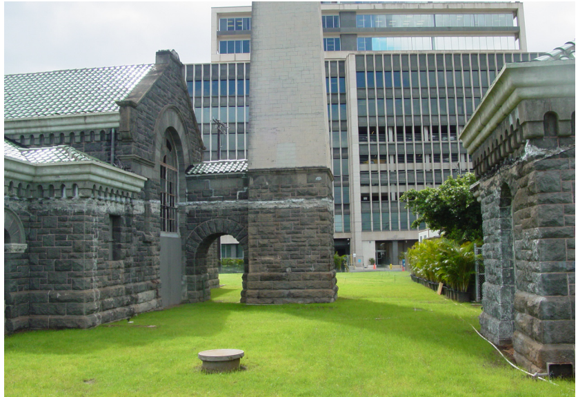
Figure 31: Current state of Ewa side of 1900 Pumping Station looking toward Keawe Street indicating remaining paint and waterproofing in exterior historic stone. Plywood barricades over existing openings painted gray. Capped piping in foreground. Temporary grass over concrete in foreground courtesy of HAF in association with Louis Vuitton.
