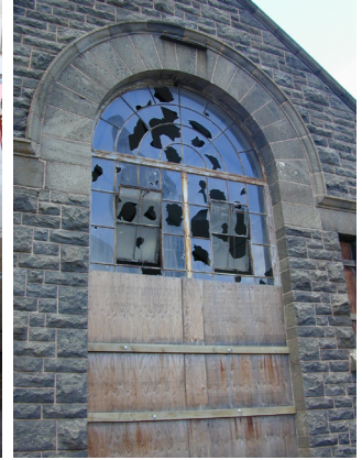
Figure 24: Extent of broken windows and deteriorated frames prior to the removal of the plywood and the addition of a temporary sheet of plexiglass on the interior face.
