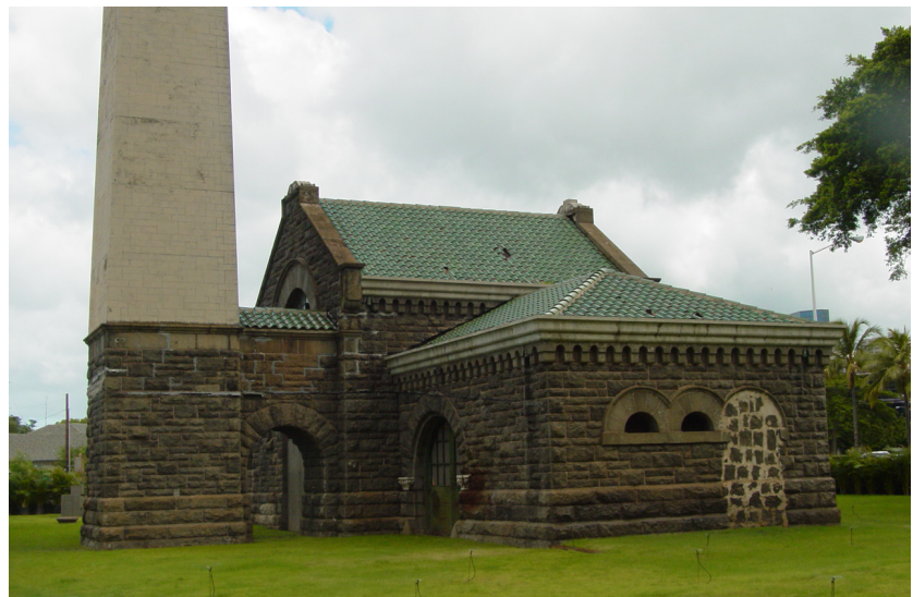
Figure 32: Closeup of Diamond Head side facing Forrest Avenue. Note section of window and wall that should be restored on right. Concrete slab in front of archway on left has been temporarily grassed and should be removed.
