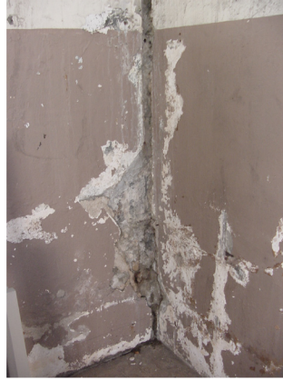
Figure 23: Damaged and settling plaster interior walls of the 1900 Pumping Station. The abandoned electrical conduit has been removed by the HAF in association with Louis Vuitton.
