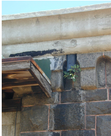
Figure 29: Damage to cornice and missing downspouts, typical. Wood structure to left removed by HAF.
