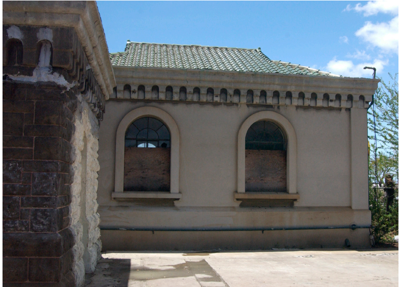
Figure 35: 1939 Pump House with broken glazing and concrete in foreground under temporary grass landscaping.
