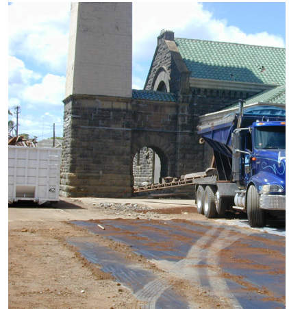
Figure 27: Remaining concrete foundation in front of archway that was covered with temporary grass landscaping.
