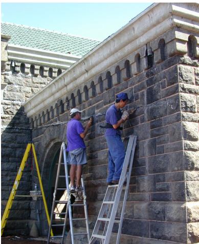
Figure 28: HAF volunteers removing some of roof waterproofing from historic structure.
