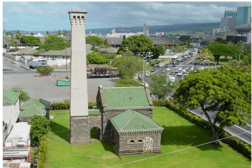
Figure 33: Current state of Diamond Head side of building looking toward Forrest Avenue. Vacant Forrest Avenue parcel in background. Gray painted plywood cover over access pit to 1939 suction chamber can be seen just behind the Screen House on the left.
