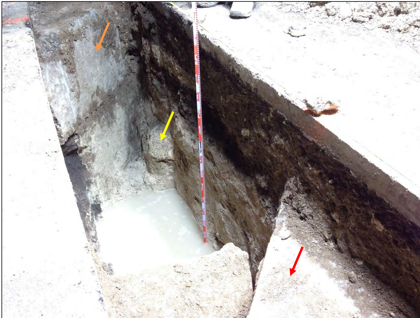
Figure 97. Photograph of the TE 15 northeast sidewall, view to north; note the structural grade beam (orange arrow), limestone boulders (SIHP # -7655, Feature 1) (yellow arrow), and the concretized Ward Estate 'auwai (SIHP # -7659) (red arrow)
