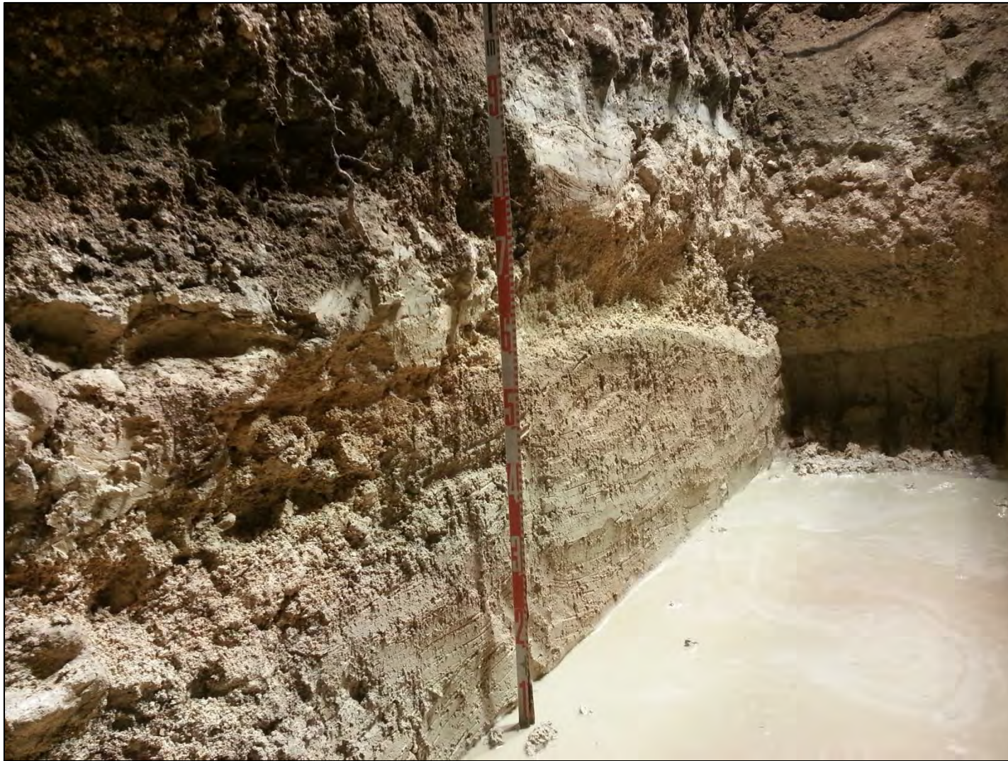
Figure 175. Close-up of the man-made berm (SIHP # -7655) (Stratum II) within the TE 35 southwest sidewall, view to southwest
