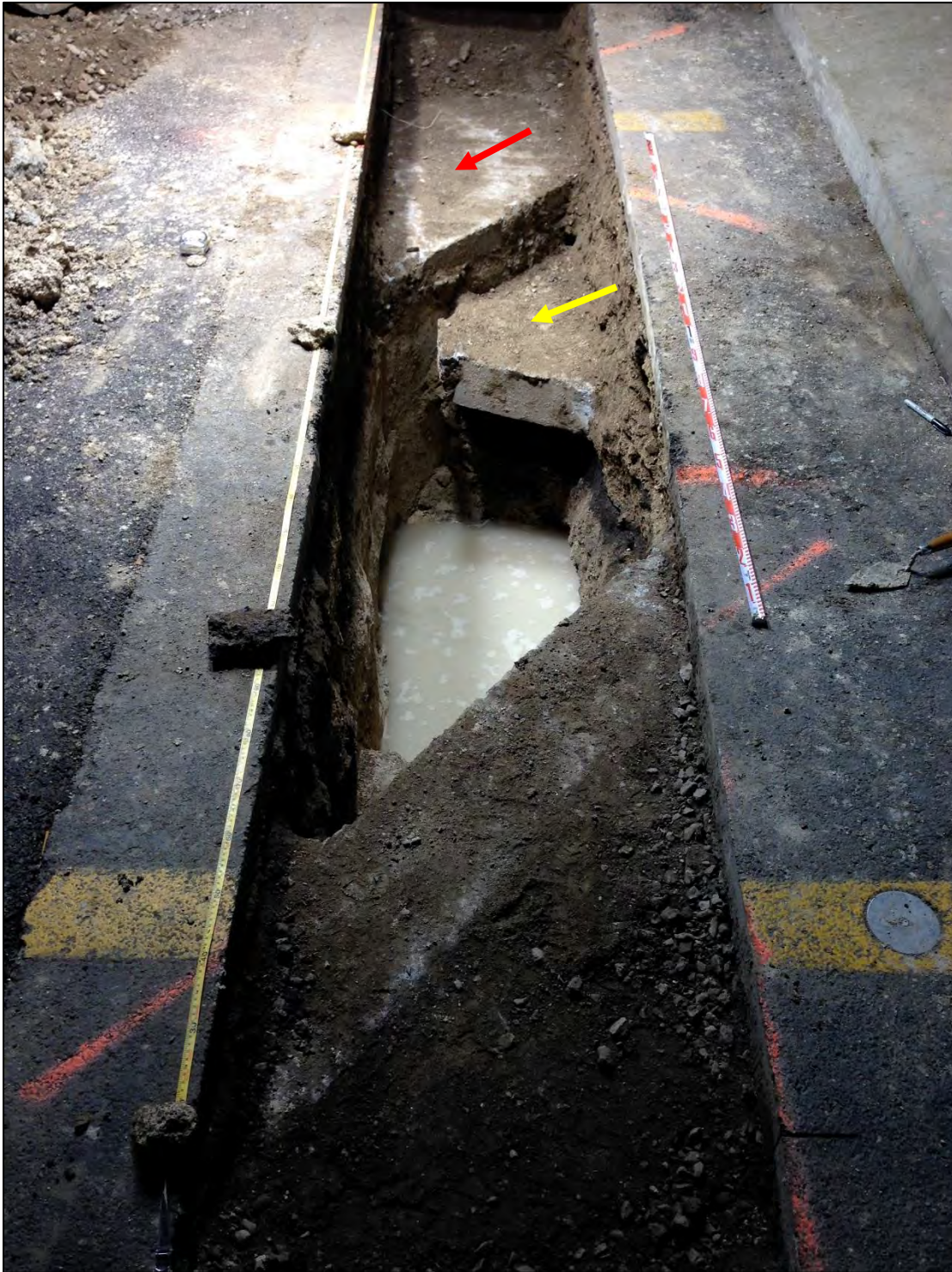
Figure 98. Overview of the Ward Estate 'auwai (SIHP # -7659) (red arrow) located at the far end of the test excavation, and the adjacent concrete slab (yellow arrow) placed to protect the existing utility
