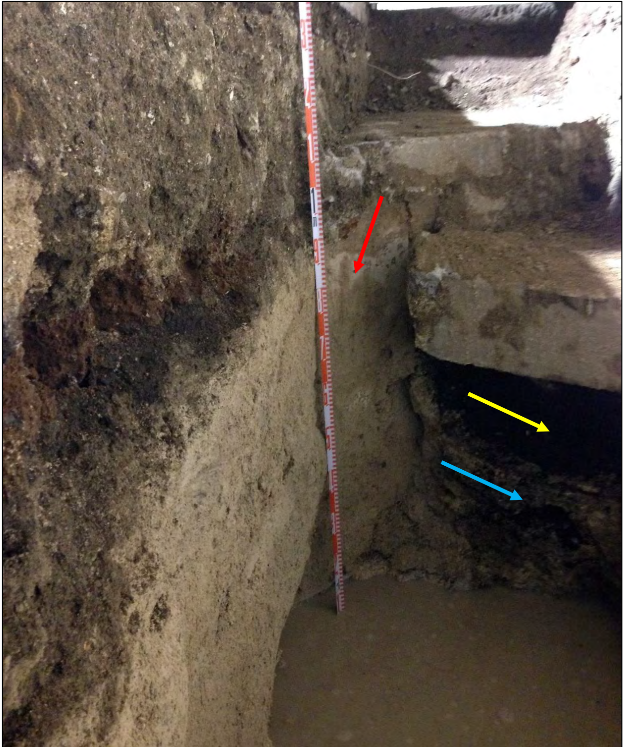
Figure 99. Close-up of the Ward Estate 'auwai (SIHP # -7659) (red arrow) showing the opening through the 'auwai for the existing utility (yellow arrow) and the retainment buffer extending to 40 cm above the coral shelf (blue arrow)
