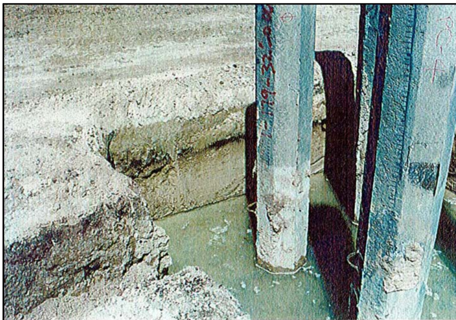
Figure 38. Photograph of pile cap trench showing old A horizon (dark stratum) capping sandy clay pond sediments (Winieski and Hammatt 2001)
