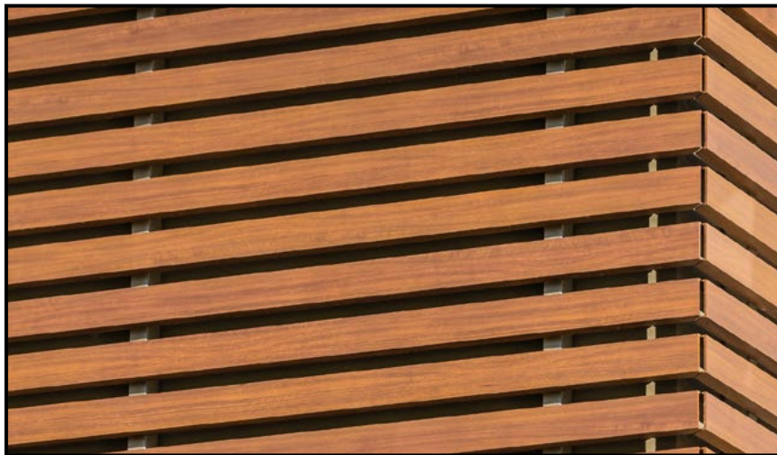
Example of metal composite installation
