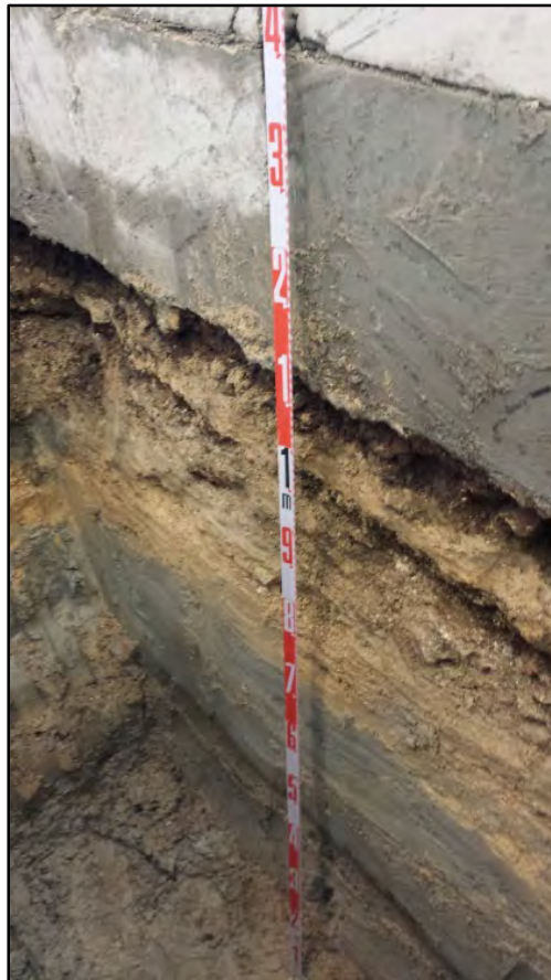
Figure 186. T-33 southeast sidewall, view to east
