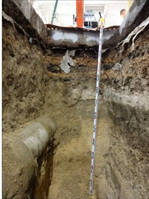
Figure 147. T-24 southwest wall showing a utility line extending along the southeast sidewall, view to southwest
