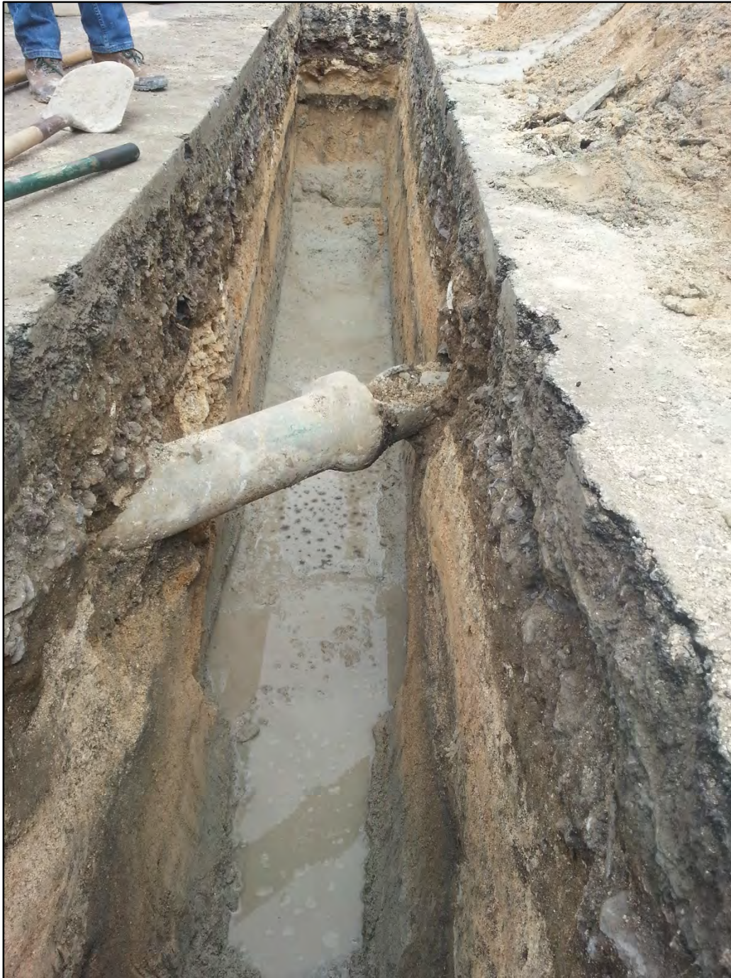
Figure 57. Photograph of T-2, showing both sidewalls
