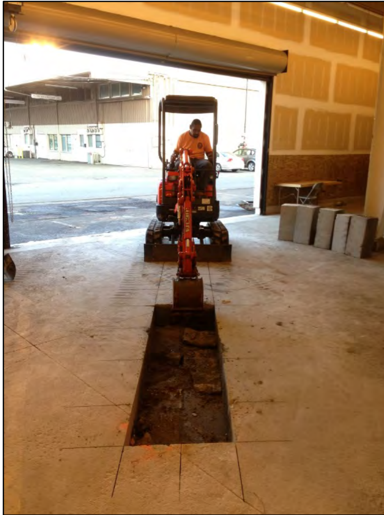
Figure 75. Location of T-7 within the loading dock of the former Nordstrom Rack building, showing removal of the thick concrete loading dock slab
