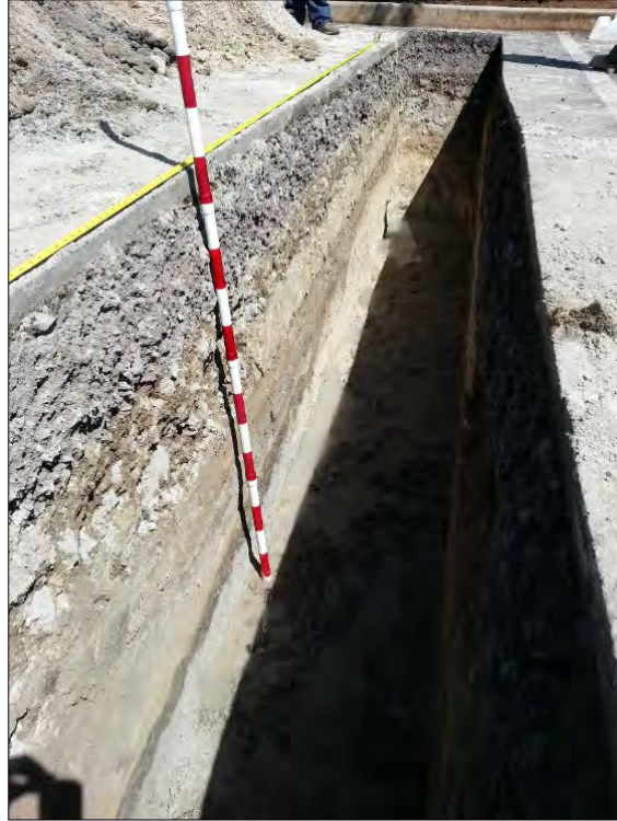
Figure 243. T-52 northwest wall, view to north
