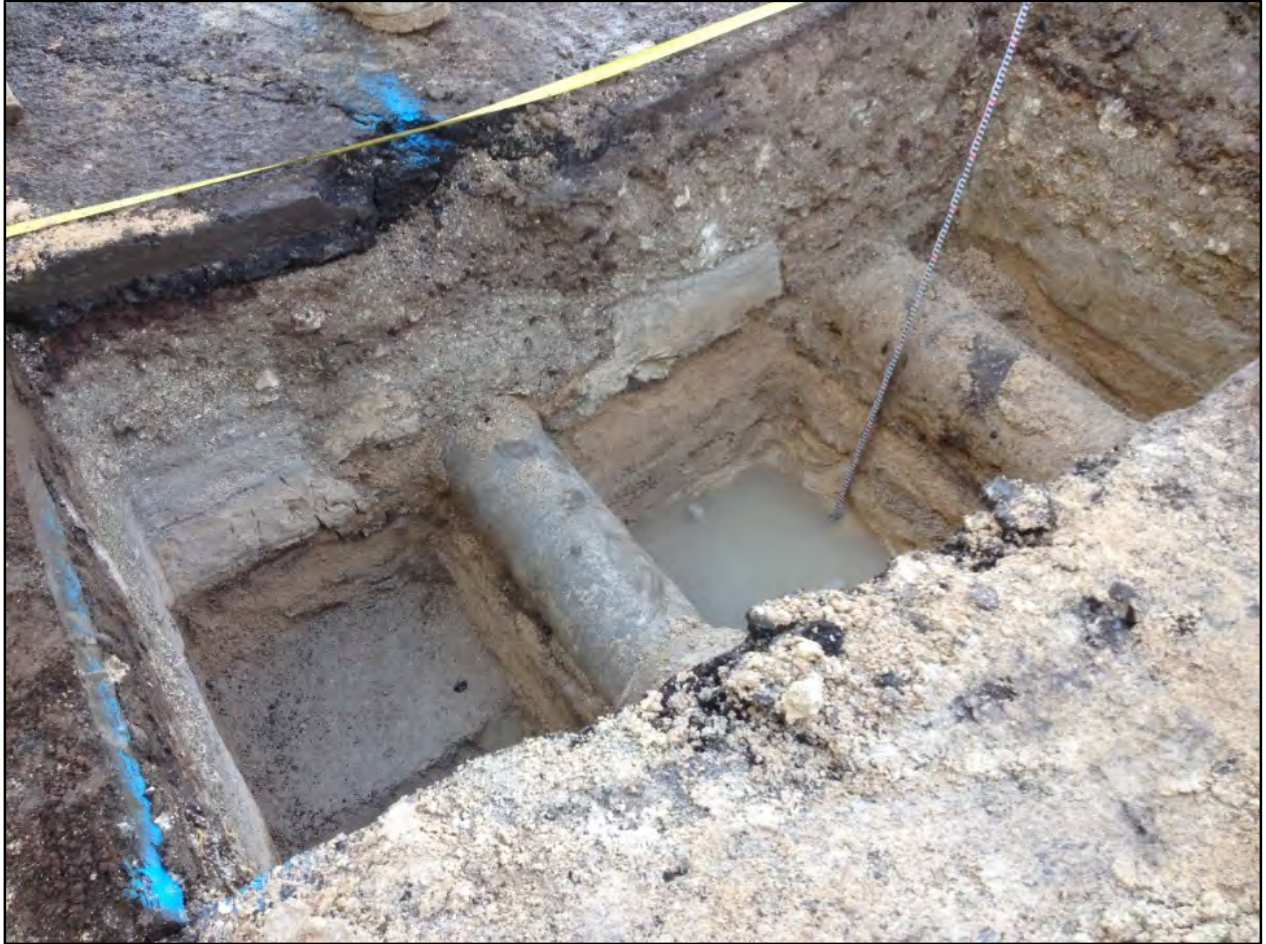
Figure 121. Photograph of T-18 northwest wall, view to north
