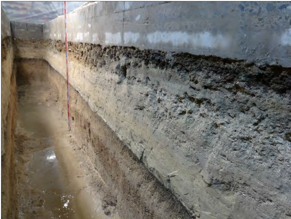
Figure 194. T-35 southeast wall, view to north
