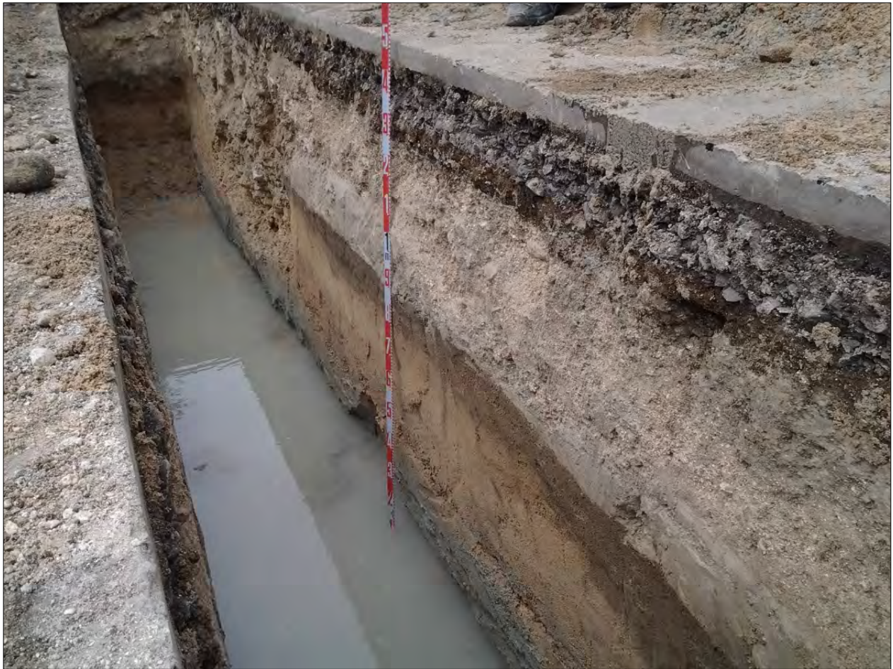
Figure 63. Photograph of T-3 northwest wall, view to southwest
