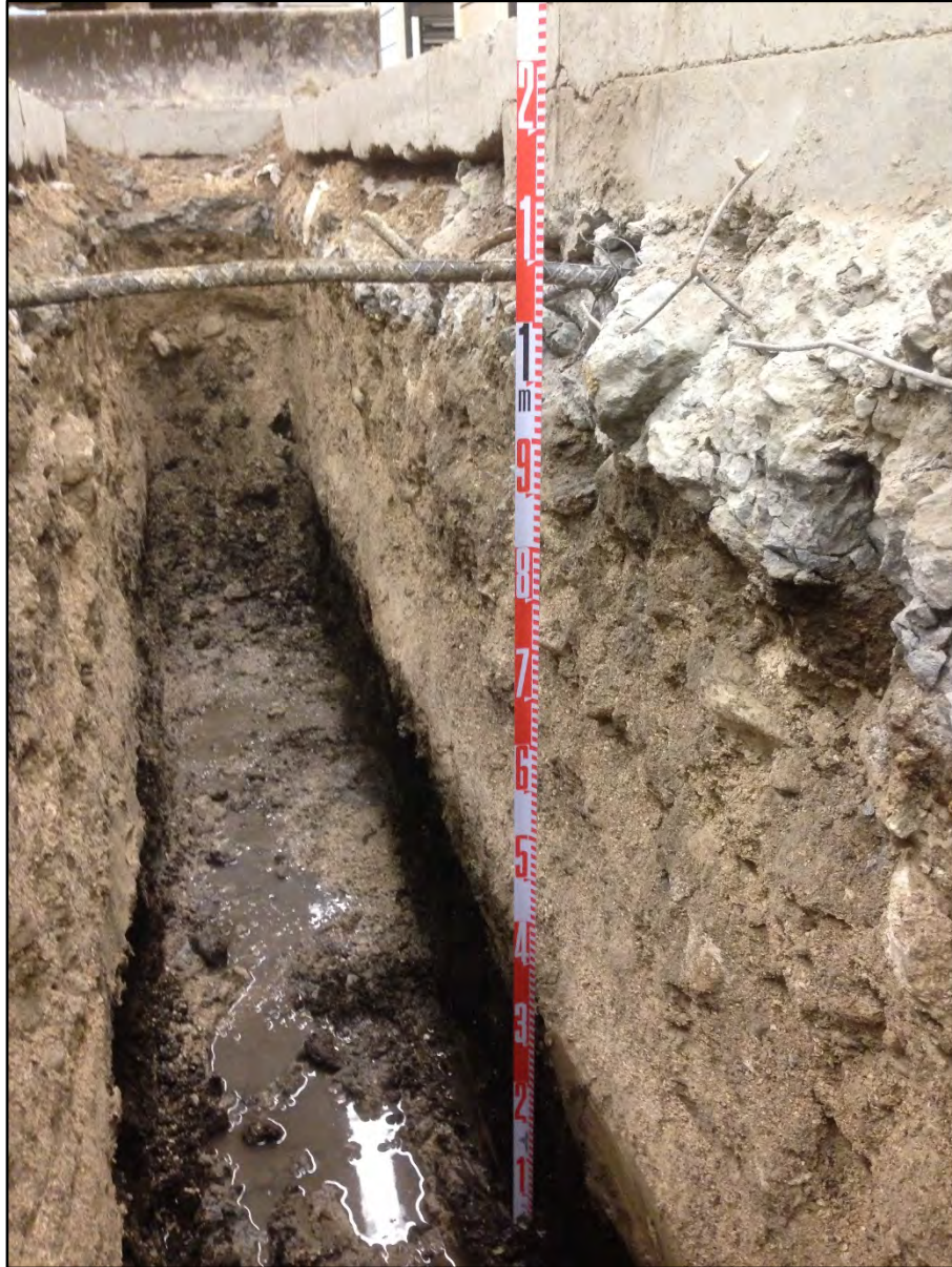
Figure 105. Photograph showing multiple concrete surfaces consisting of the current commercial floor (Stratum Ia) directly overlying an earlier concrete surface associated with SIHP # -7686 (Stratum Ic), overlying an additional buried concrete surface containing rebar and wire (Stratum Id) (SIHP # -7686)
