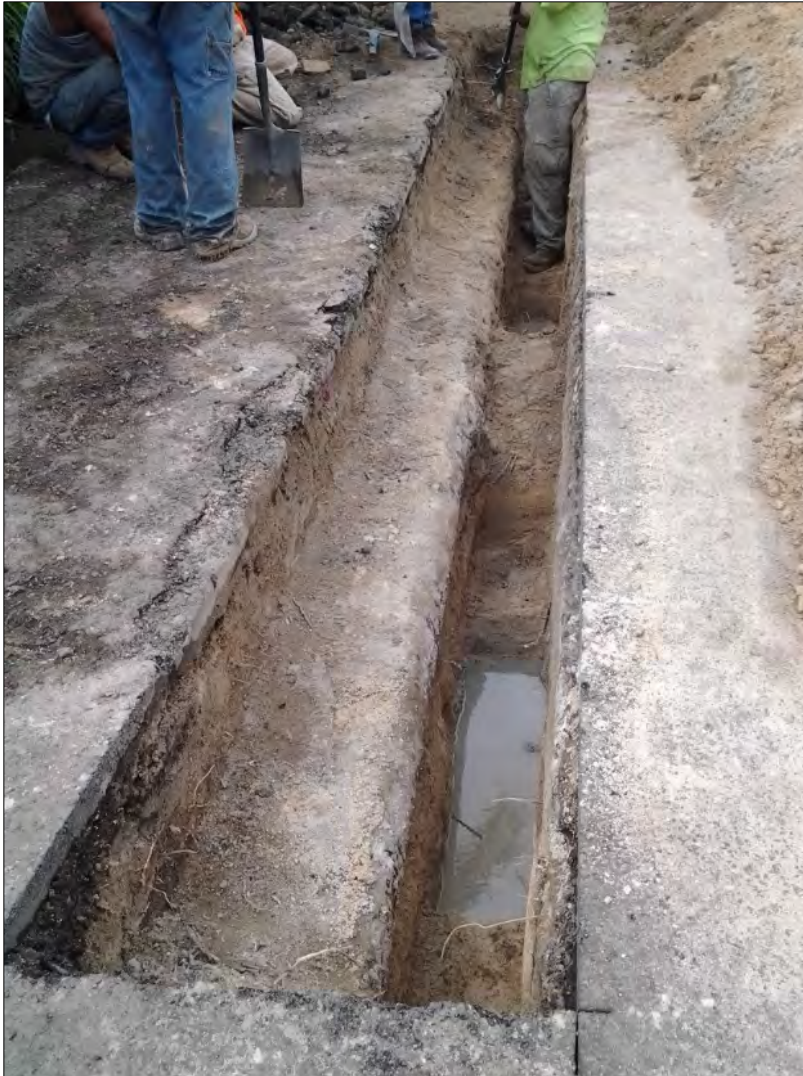
Figure 198. Photograph showing utility running parallel with the south wall, view to northwest
