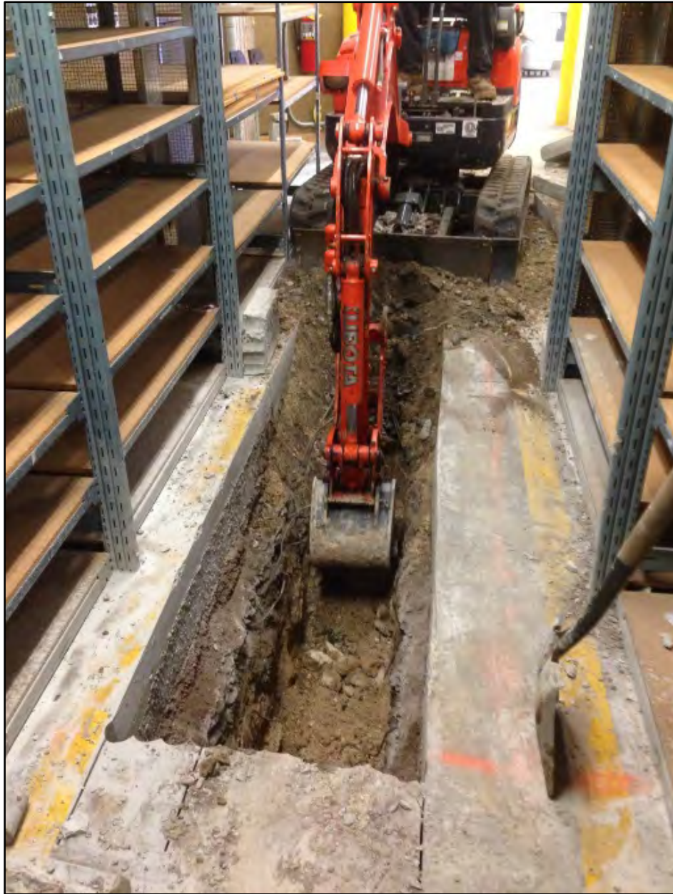
Figure 98. Location of T-13 within the back storage area of a commercial establishment
