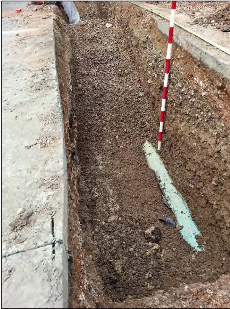
Figure 263. T-58 northeast wall with base course fill material and utility pipes, view to north
