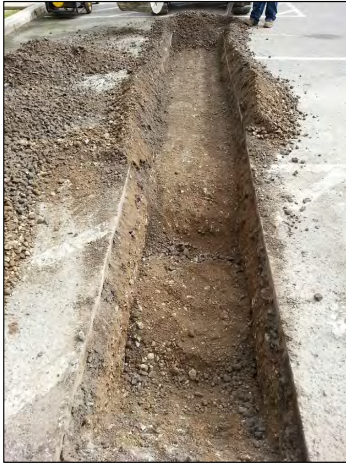
Figure 200. T-37, post excavation, view to northeast
