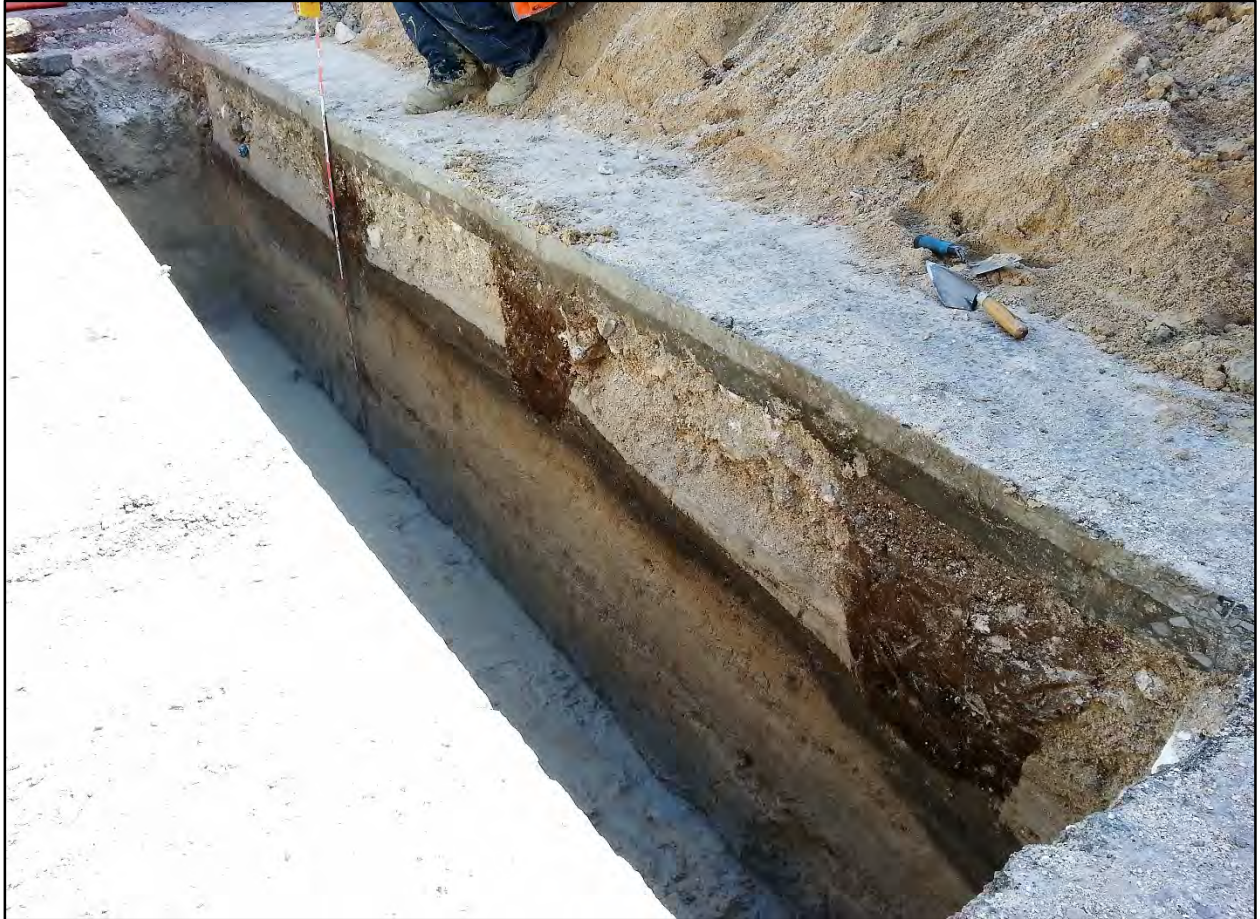
Figure 305. T-68 southwest wall, view to west
