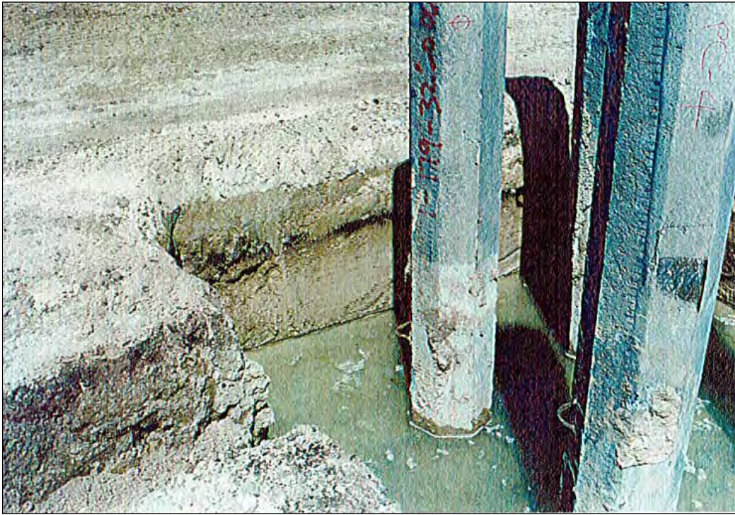
Figure 40. Photograph of pile cap trench showing old A horizon (dark stratum) capping sandy clay pond sediments (Winieski and Hammatt 2001)
