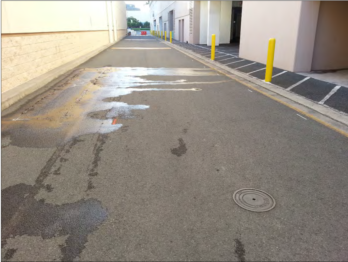
Figure 95. Location of T-12 within the alleyway between the Ward Theaters and the former Nordstrom Rack building, view to southeast
