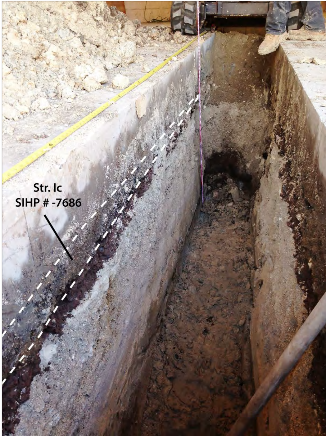
Figure 365. Photograph of the asphalt (SIHP # -7686) and associated base course within T-7 east wall
