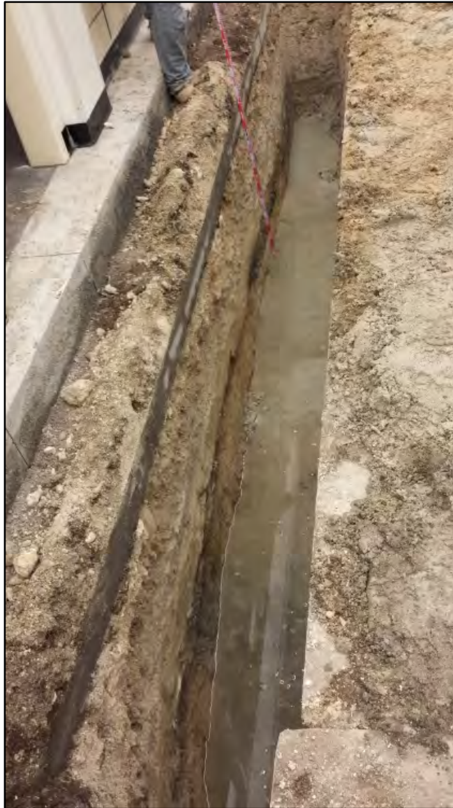
Figure 107. T-15 northwest wall, view to north
