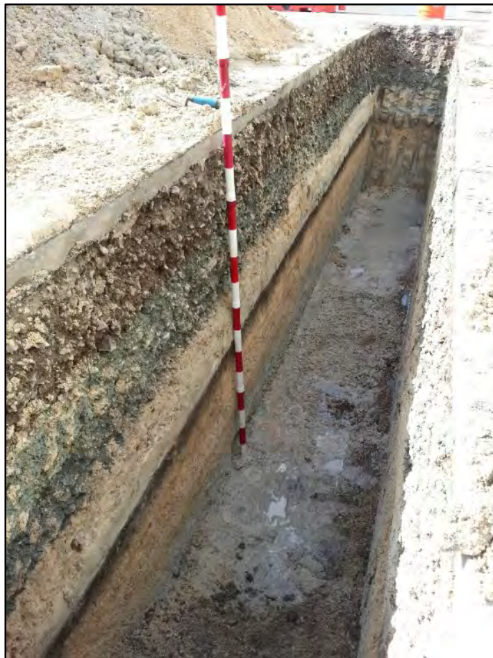
Figure 234. T-49 southwest wall, view to west
