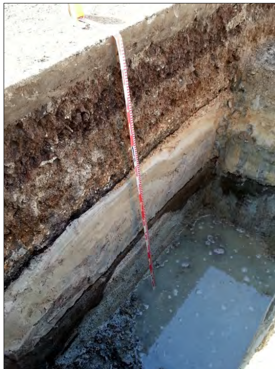
Figure 257. T-56 southeast wall ( makai end), close-up of the Stratum IIIa abrupt and irregular lower boundary, view to south
