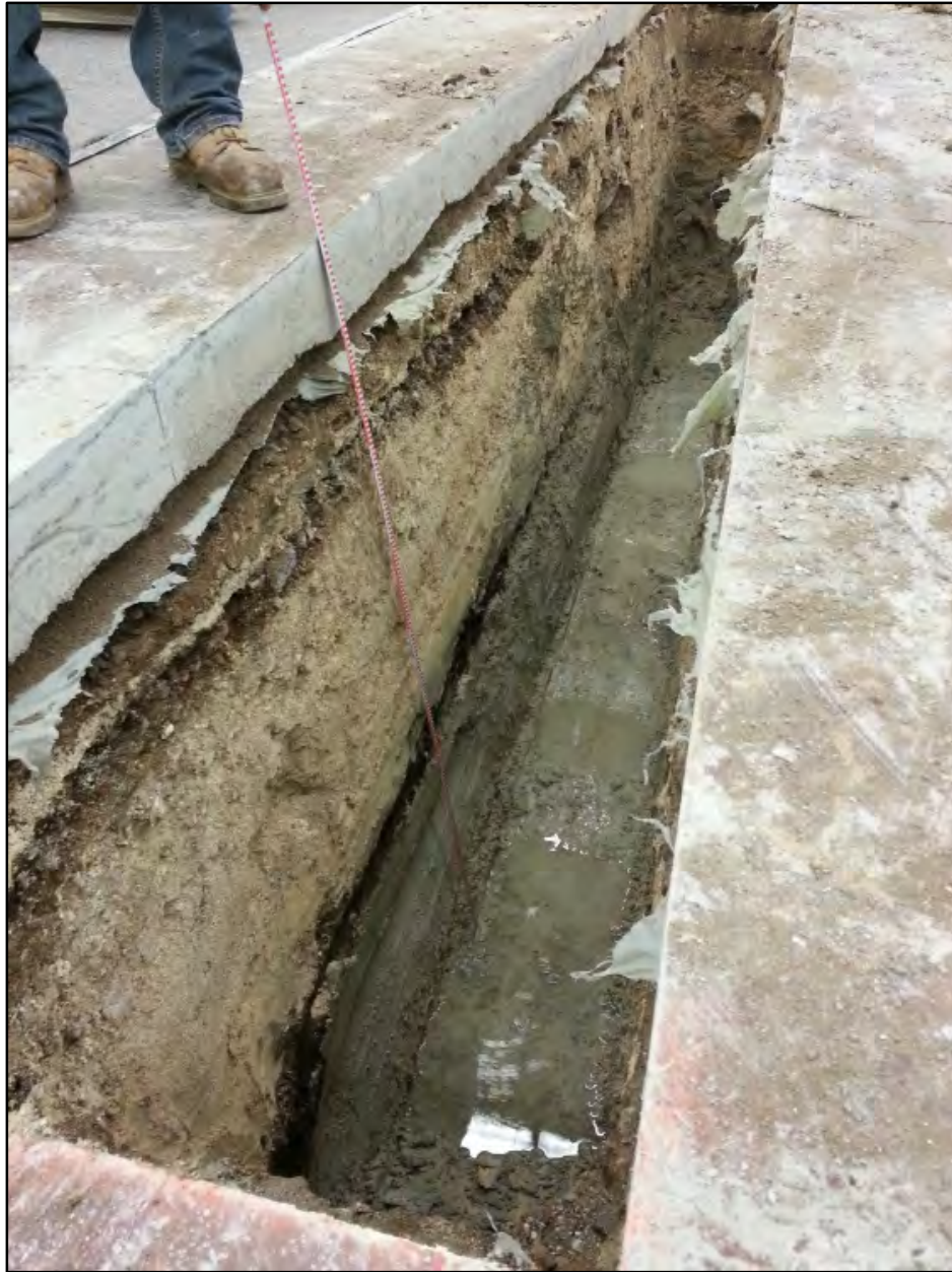
Figure 130. T-21 north wall, view to north
