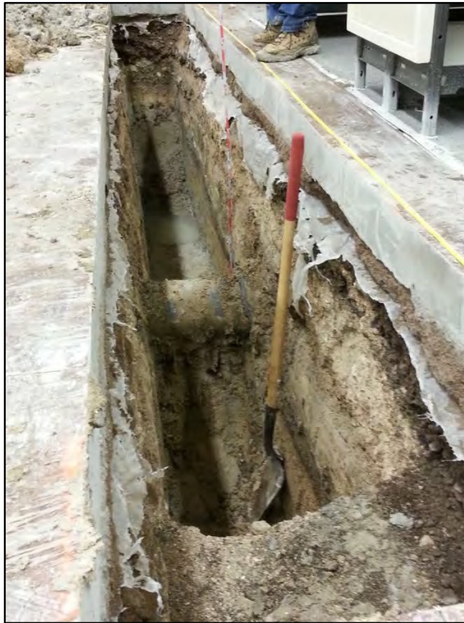
Figure 123. T-19 southwest wall, view to south
