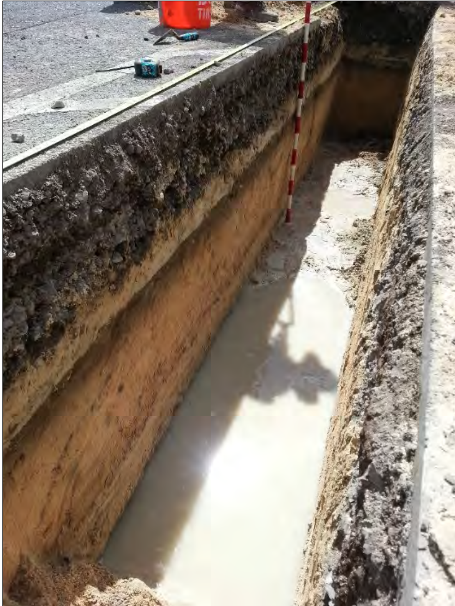
Figure 218. T-43 southeast wall, view to south
