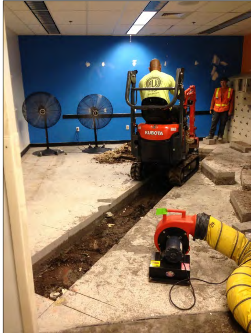
Figure 82. Location of T-9 within the back room of the former Nordstrom Rack commercial store
