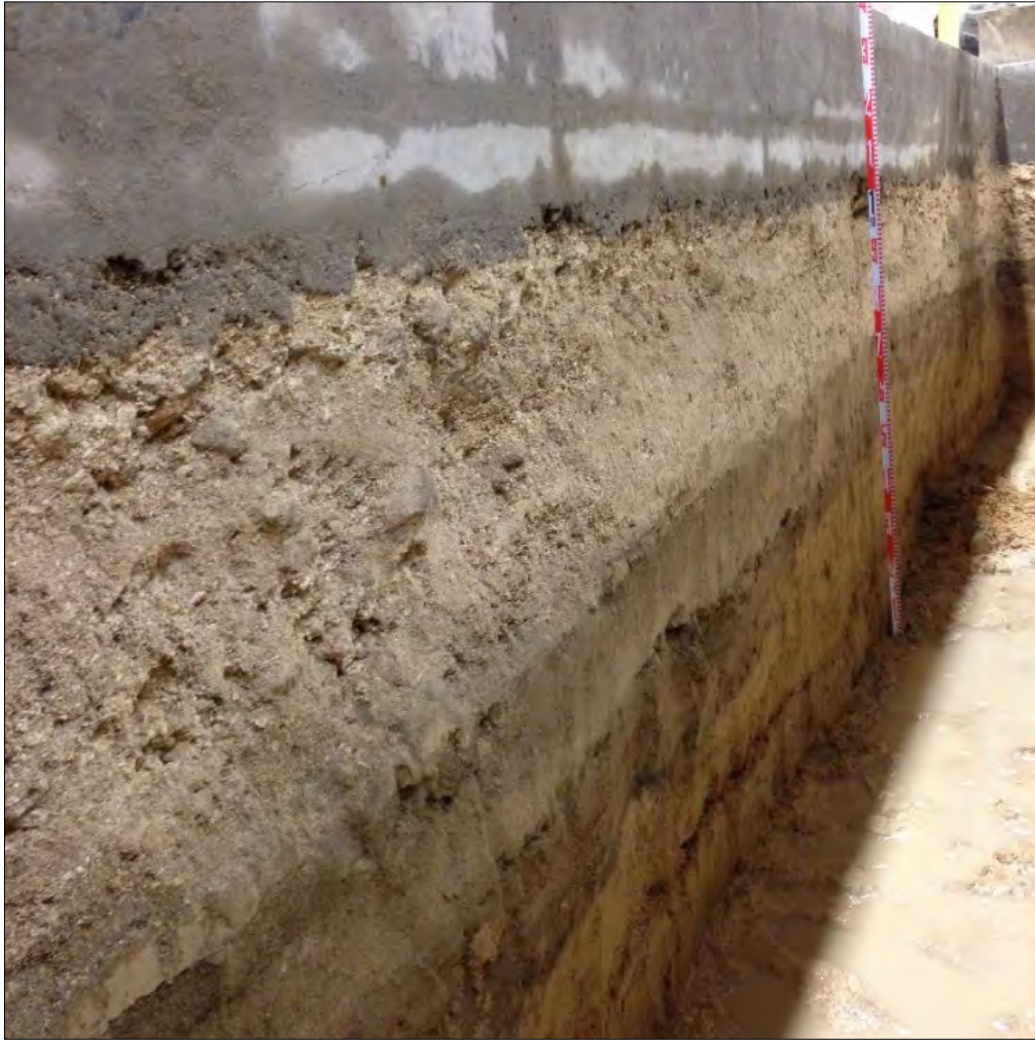
Figure 137. Photograph of T-23 northwest wall, view to north
