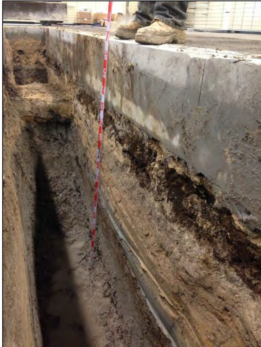
Figure 127. T-20 southwest wall, view to south
