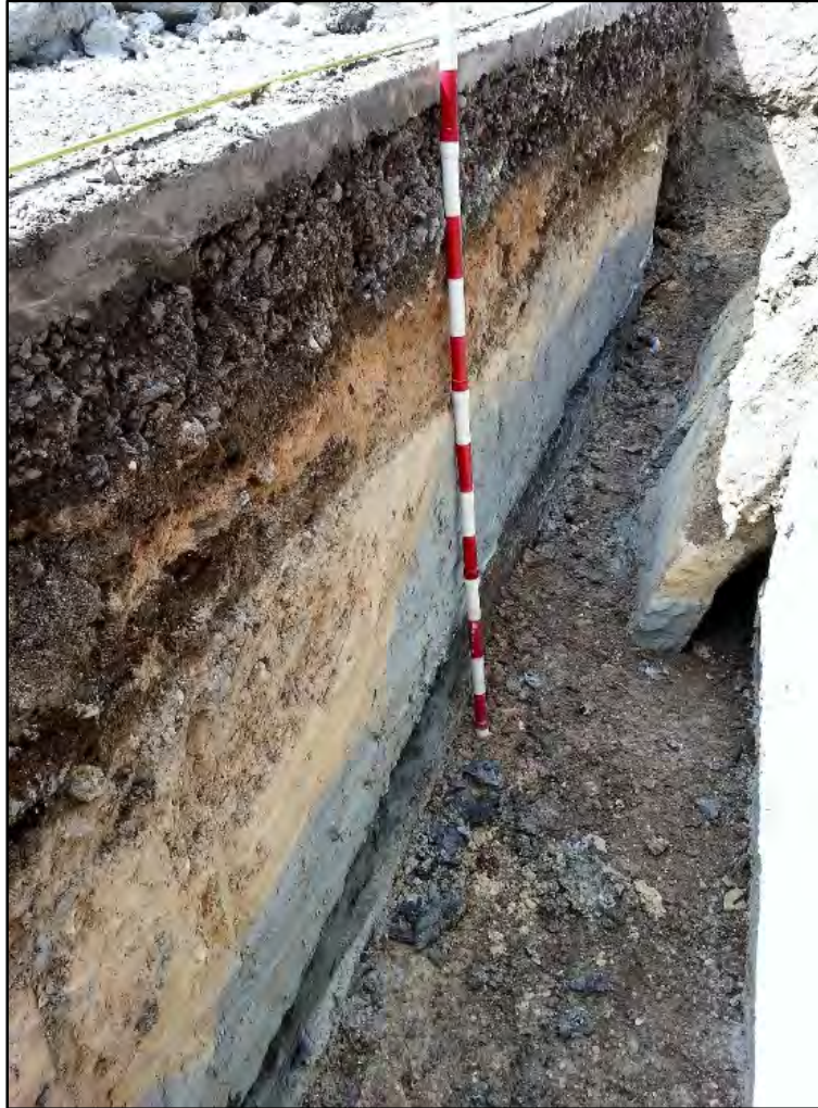
Figure 268. T-60 southwest wall, showing collapse of the northeast wall, view to west
