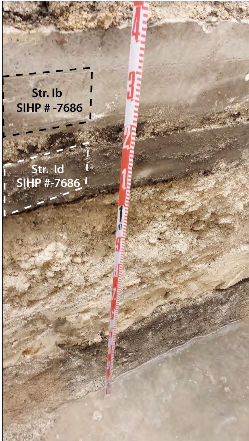
Figure 360. Photograph of the multiple buried concrete surfaces (SIHP # -7686) with associated base courses within the T-15 southeast wall
