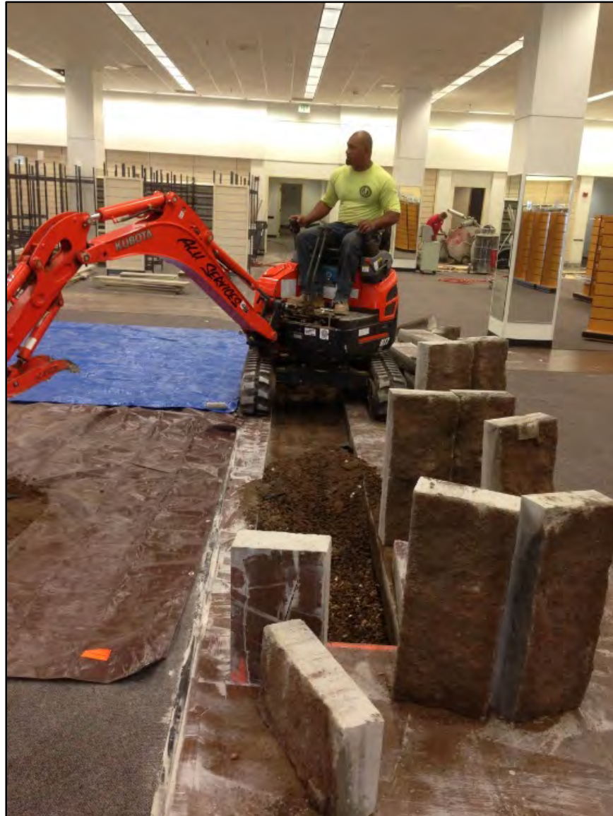
Figure 132. Location of T-22 within interior commercial space, view to northwest
