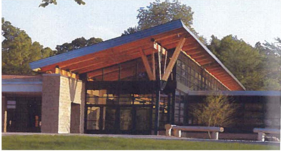
SLOPE ROOF AND DAYLIGHTING
