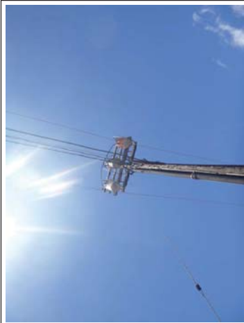
Photograph 3: Non-PCB HECO transformers that appeared to be rusting.
