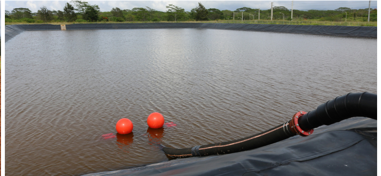
A new pumping system will transport irrigational water from our property reservoirs.
