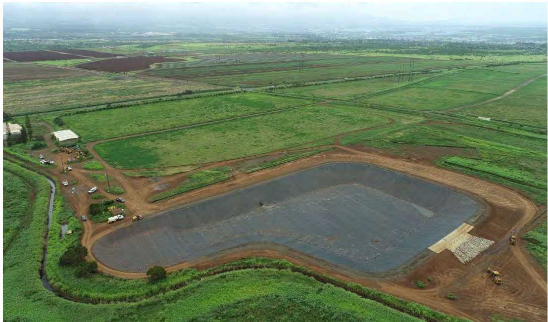
15 MGD Reservoir, Kunia, Oahu
