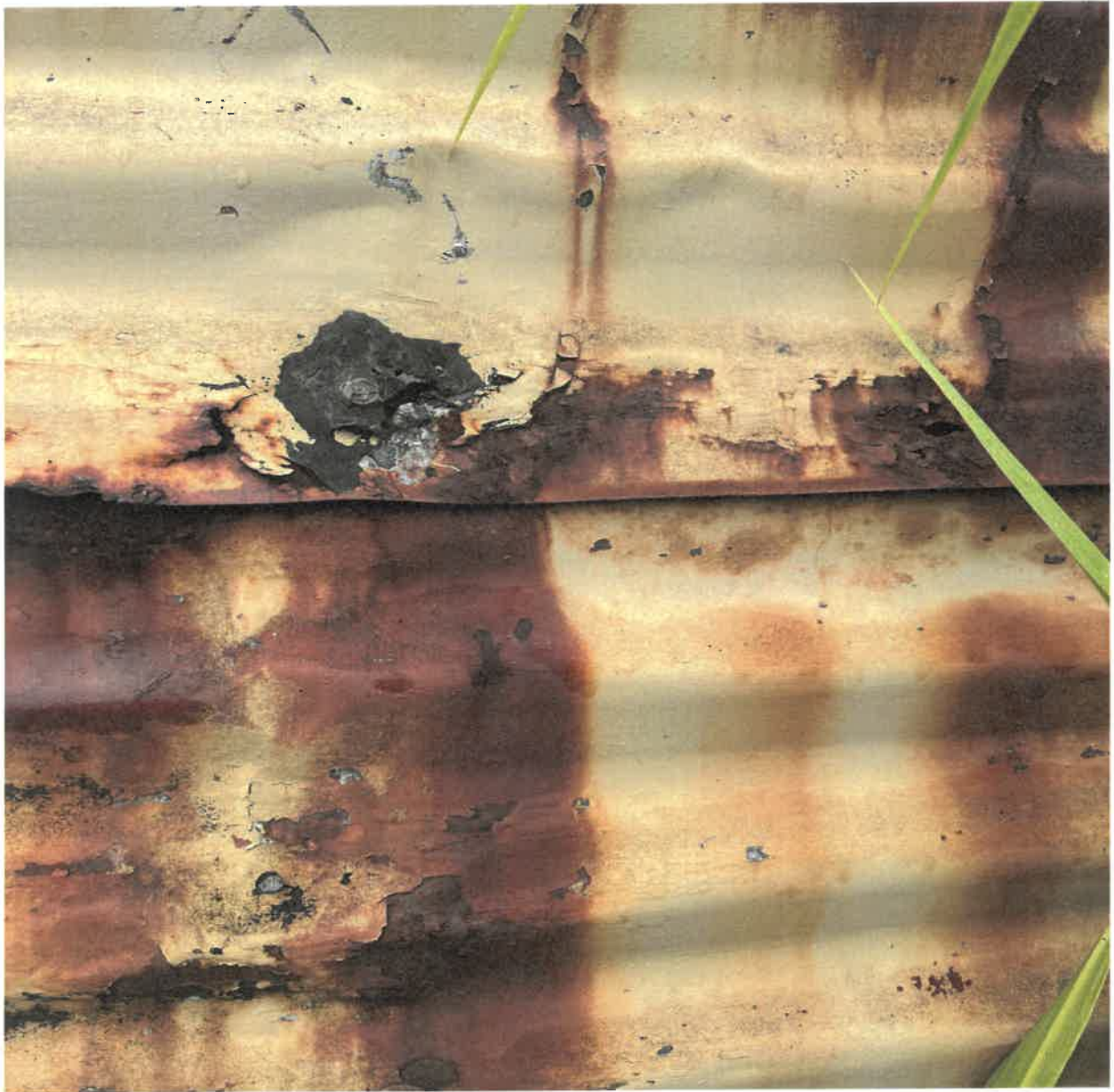
QUNNSET HUT EXTERIOR PANELS (BLACK CAULKING/SEALANT)
