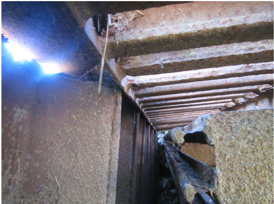
Photo 4 – Sheet Pile Behind Mauka Abutment
