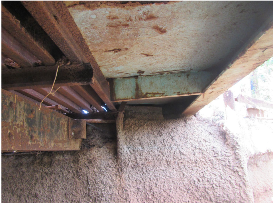
Photo 3 – Plate Extension Framing
