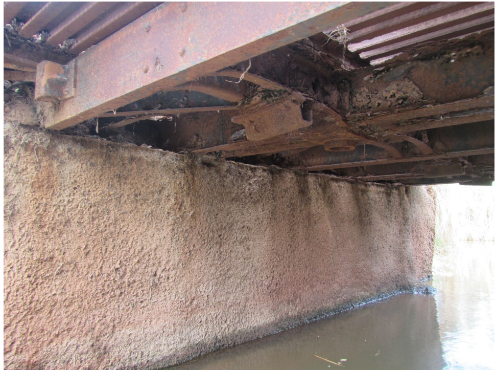
Photo 2 – Bridge from Below
