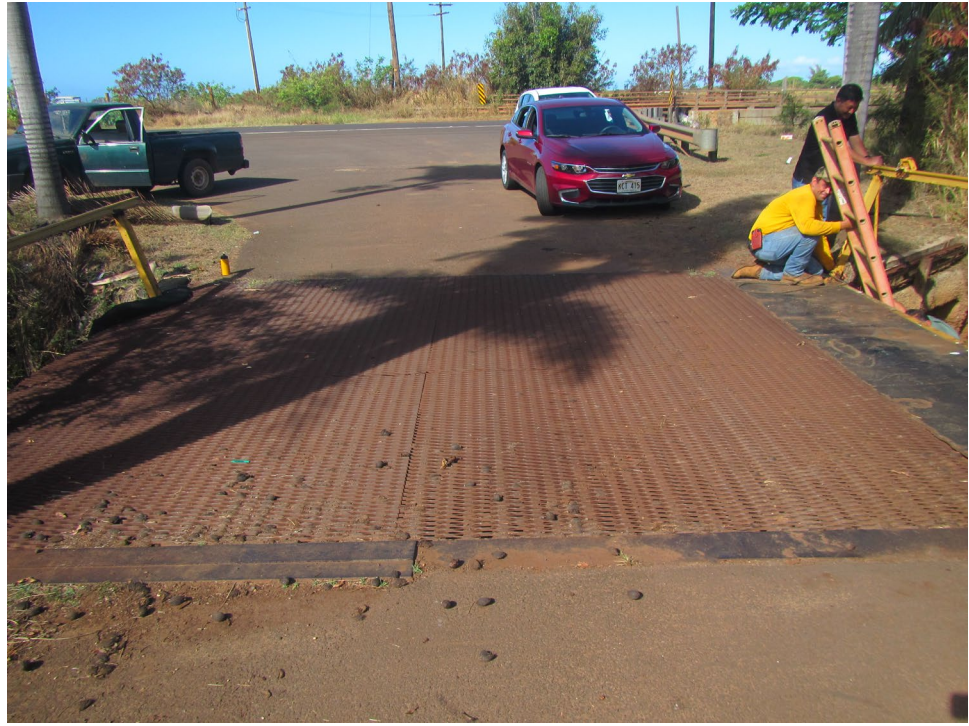
Photo 1 – Bridge from Above
