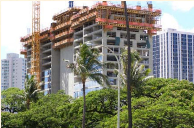
Moana Vista under construction
