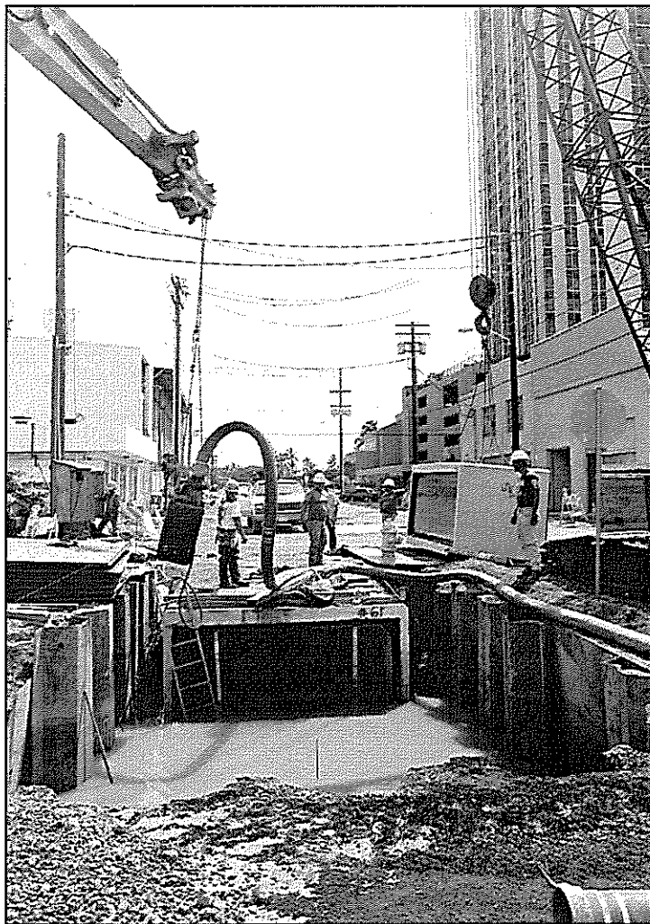
Drainage boxes are installed on Kamakee Street
