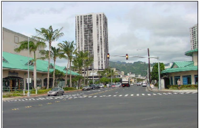
Kamakee Street after construction of infrastructure improvements.
