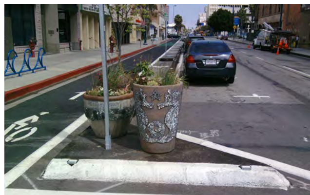
Most Complete Streets projects in KCDD will be retrofits of existing roadways, like this bikeway retrofit of Third Street in Long Beach, CA.
