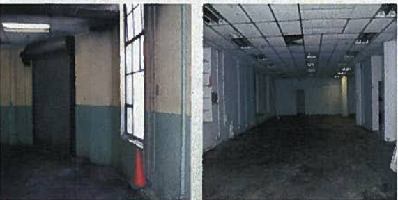
Office Space Under the Flat Roof
