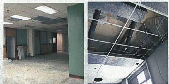
Office Space Under the Red Tile Roof
