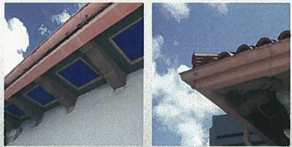
Red Tile Roof Eaves are Finished
