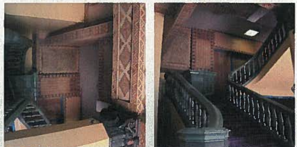
Staircase & Interior Finish
