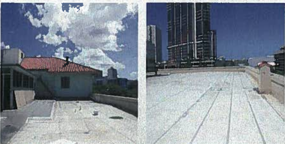
Flat Roof – Note Small Red Cupola
