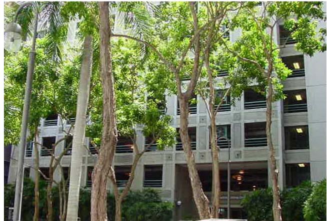
Designed to discourage visibility of parked cars from the street and rooftop. Floors visible from the street should be horizontal only; conceal ramps and ramped floors within the structure. Lights within the parking structure should be shielded from public view and visible ceilings should be painted a dark color.
