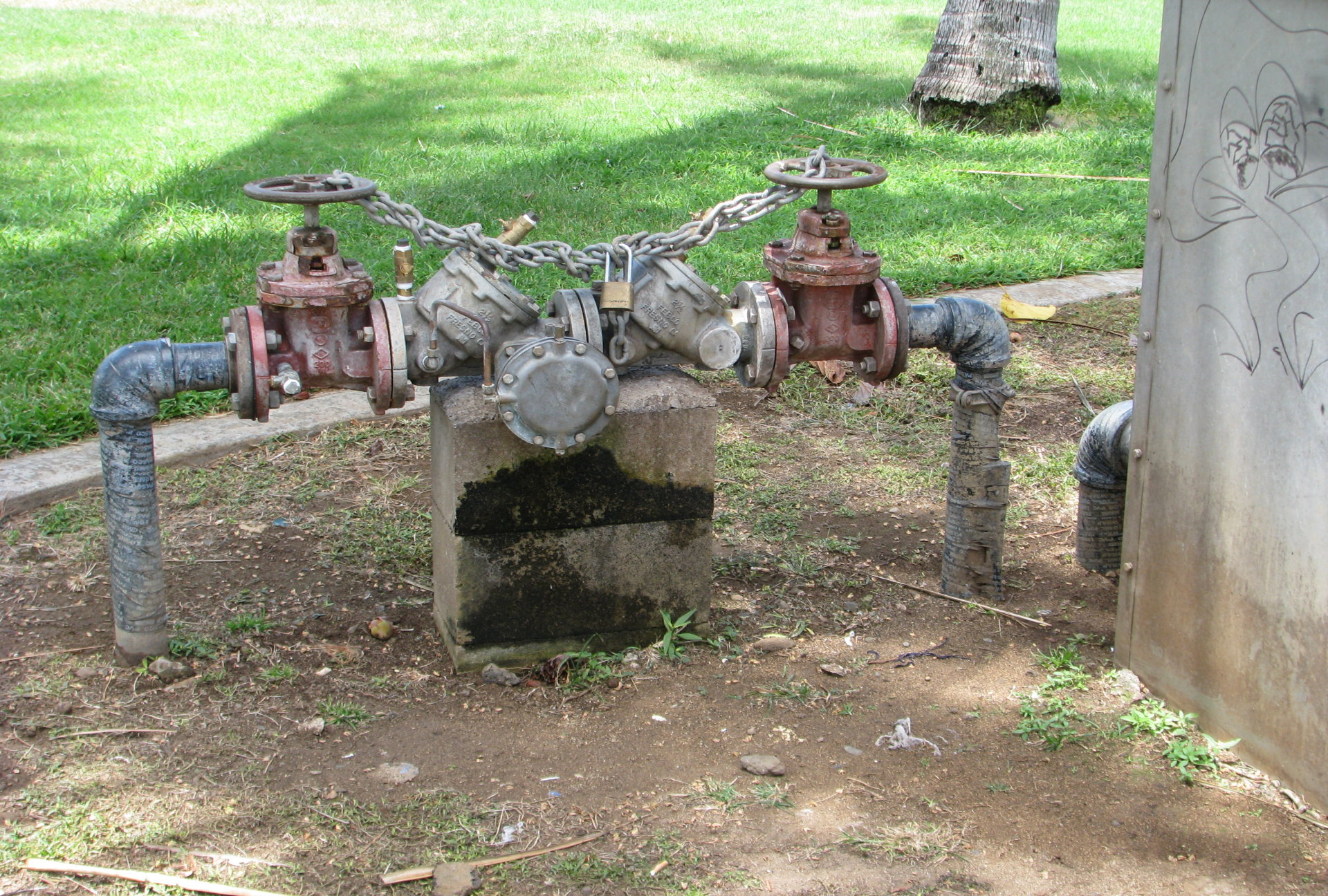
Backflow Preventers Routinely Damaged for Water Even When Boxed
