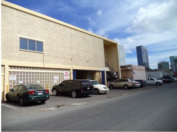
Commercial uses to west
