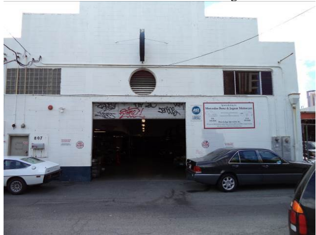
View west from Subject site toward auto repair facility
