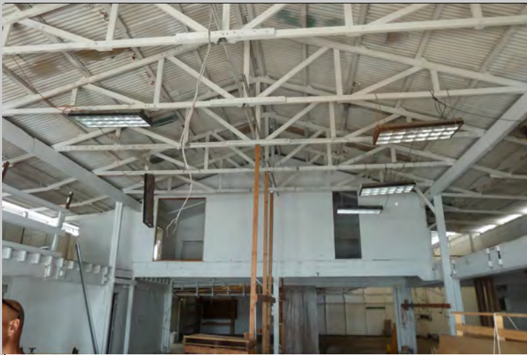
Photo 12: Interior view of vacant unit at 764 Kawaiahao Street.
