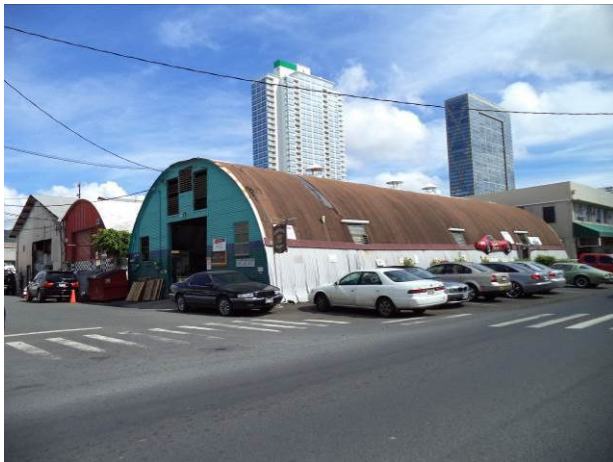
Commercial uses to west
