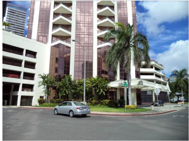
View east from Subject site toward mixed-use retail/condominium building
