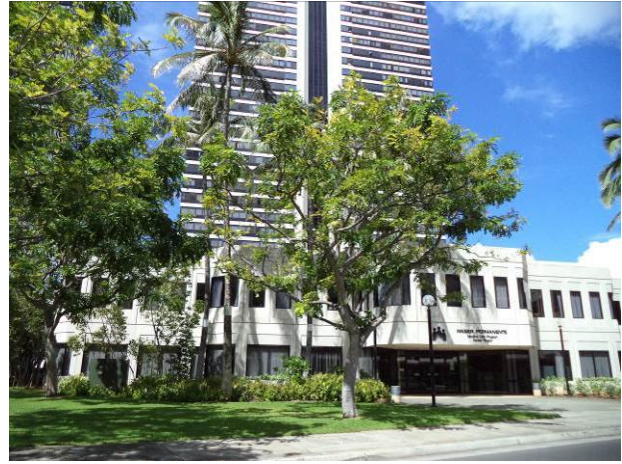
Office building to north
