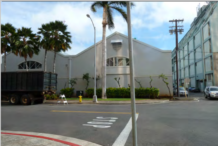
Photo 15: Adjoining property to the northeast, BMW of Honolulu.
