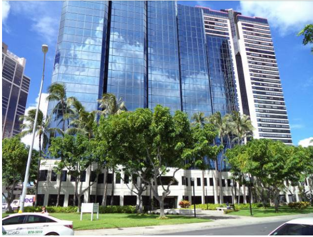
Office building to north
