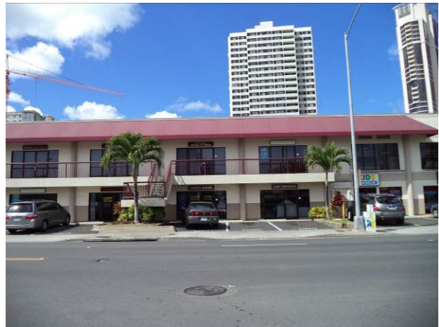
Commercial uses to west
