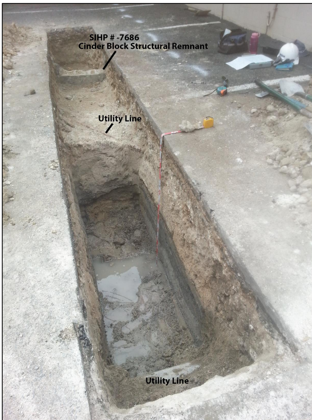
Figure 116. Block M photograph of T-1 showing a cinder block structural remnant (SIHP # -7686) and a 7-cm utility line within the makai portion of the test excavation and wetland sediments underlying modern and historic fill deposits and a utility line within the mauka portion
