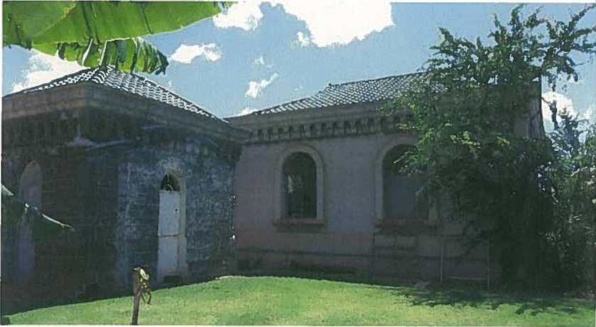
Historic Kakaako Pump Station-Built 1940 and Screen House
