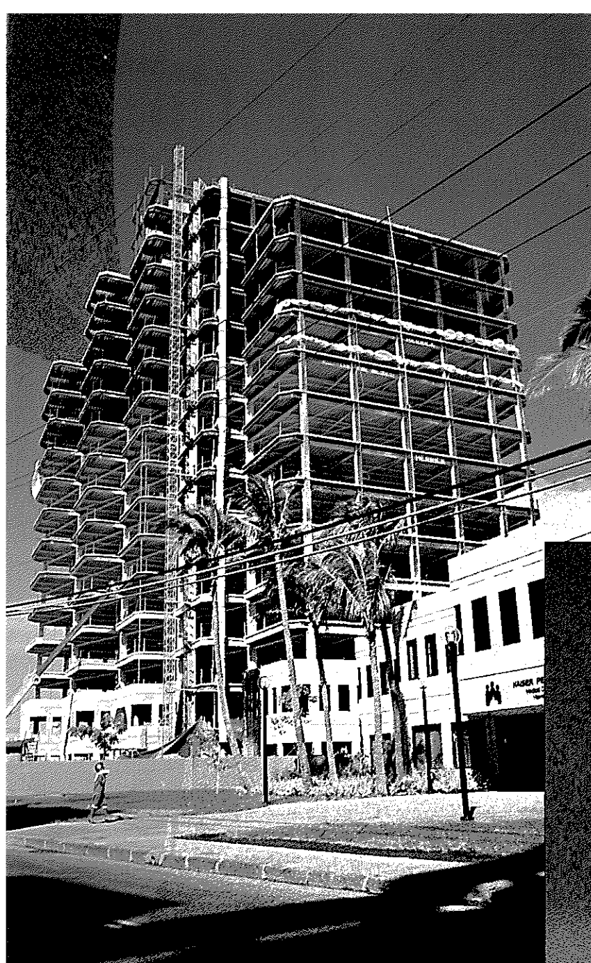
TDC Hawaii, Inc.'s commercial complex, PACIFIC PARK PLAZA, under construction.
