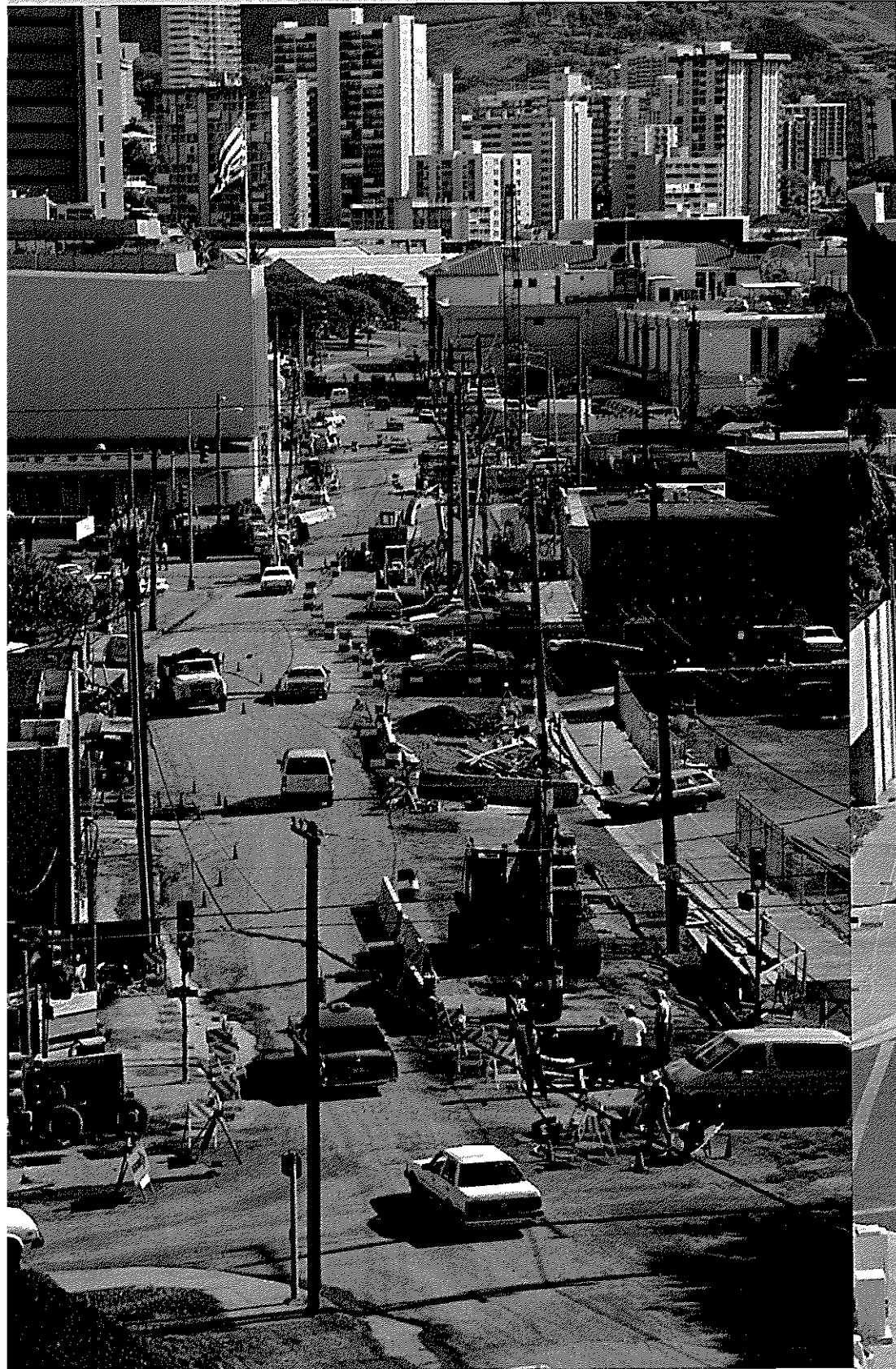
South Street during ID-1 construction.
