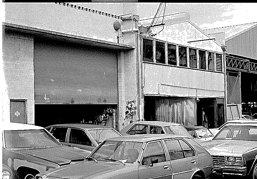
HCDA Development Director Harold Edwards (above) is seeking a solution to Kakaako's parking situation, shown at left.
