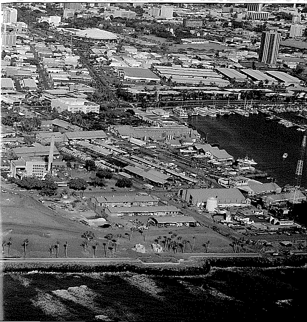
An aerial view of the Kakaako Waterfront Park now under construction.
