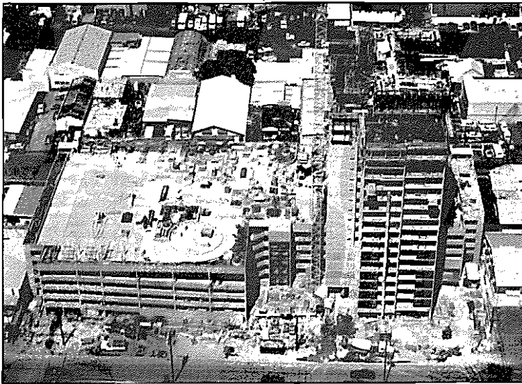
Construction of Kauhale Kaka'ako
