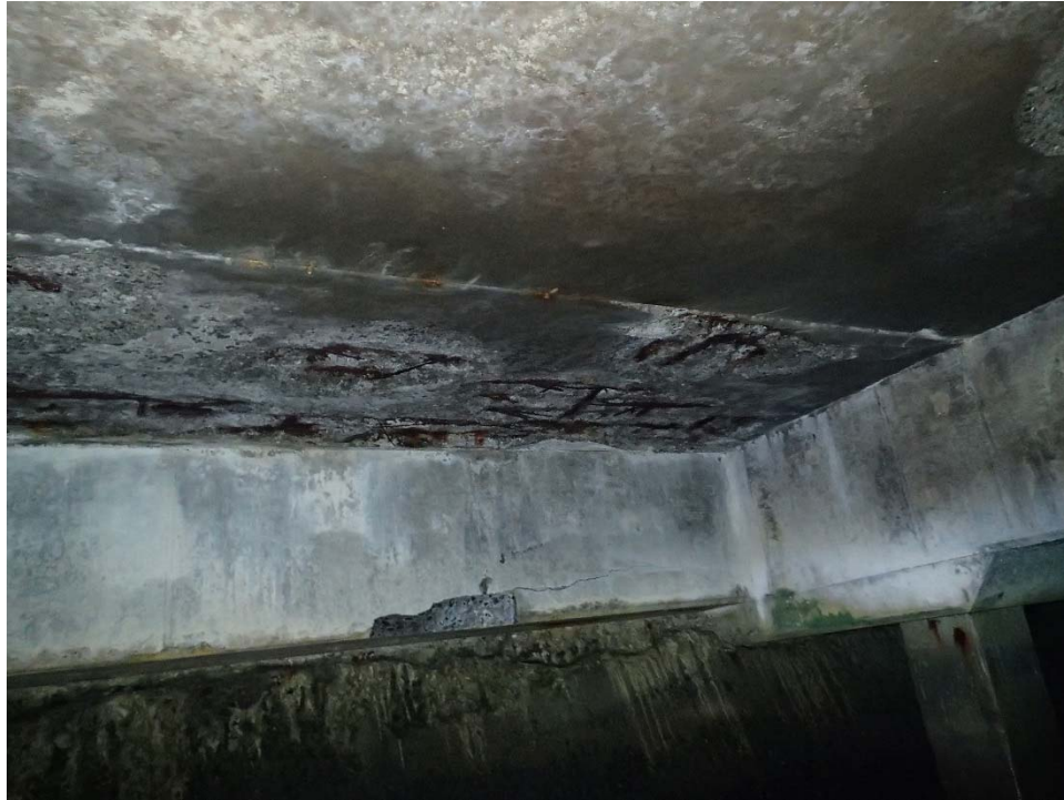
11 – Soffit of precast-prestressed plank with broken prestressing strands on the 1968 wharf
