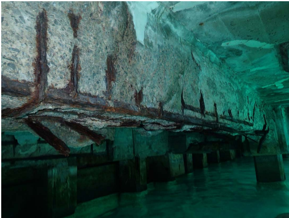
10 – Example of location with extensive beam spalling and fractured beam bottom reinforcing steel and shear stirrups on the 1924 wharf.
