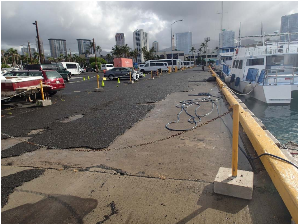
4 - Fisherman’s Wharf, looking north at the 1924 wharf construction (1968 wharf construction in foreground). Chain and posts prohibit vehicles onto the 1924 section of wharf deck.
