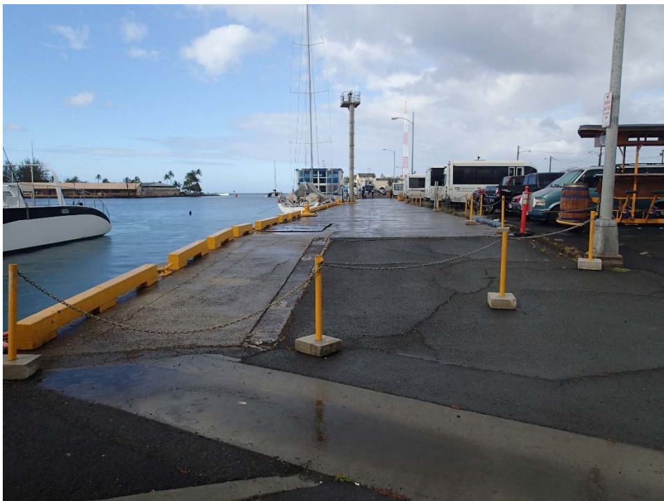
2 - Fisherman's Wharf, looking south from Ala Moana Blvd end of 1924 section of wharf. Chain and posts prohibit vehicles onto the 1924 section of wharf deck.
