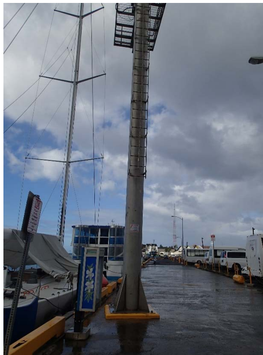
14 – 1924 section of wharf near gridline 7 with range light, telephone booth and bull rails along wharf edge
