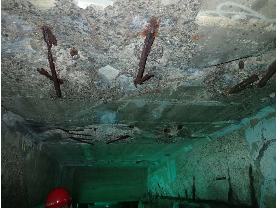
7 – Typical deck soffit and longitudinal beam damage under 1924 wharf. Note exposed and fractured slab reinforcing steel
