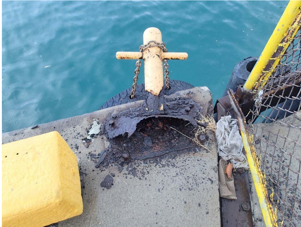
13 – Mooring cleat with significant corrosion (near collapse) at south end of 1968 wharf
