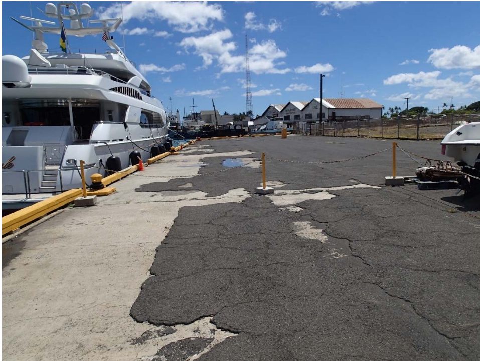
3 – Fisherman’s Wharf, looking south at the 1968 wharf construction (1924 wharf construction in foreground). Chain and posts prohibit vehicles onto the 1924 section of wharf deck.
