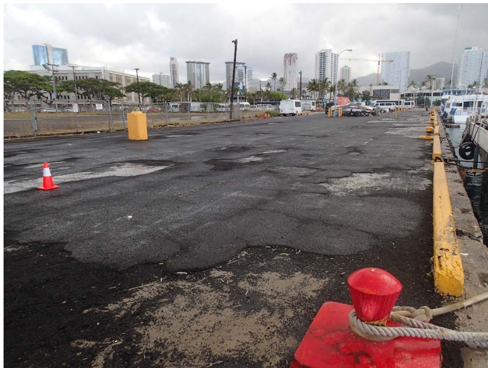
6 – Fisherman's Wharf, looking north from end of 1968 wharf. Note poor condition of asphalt topping
