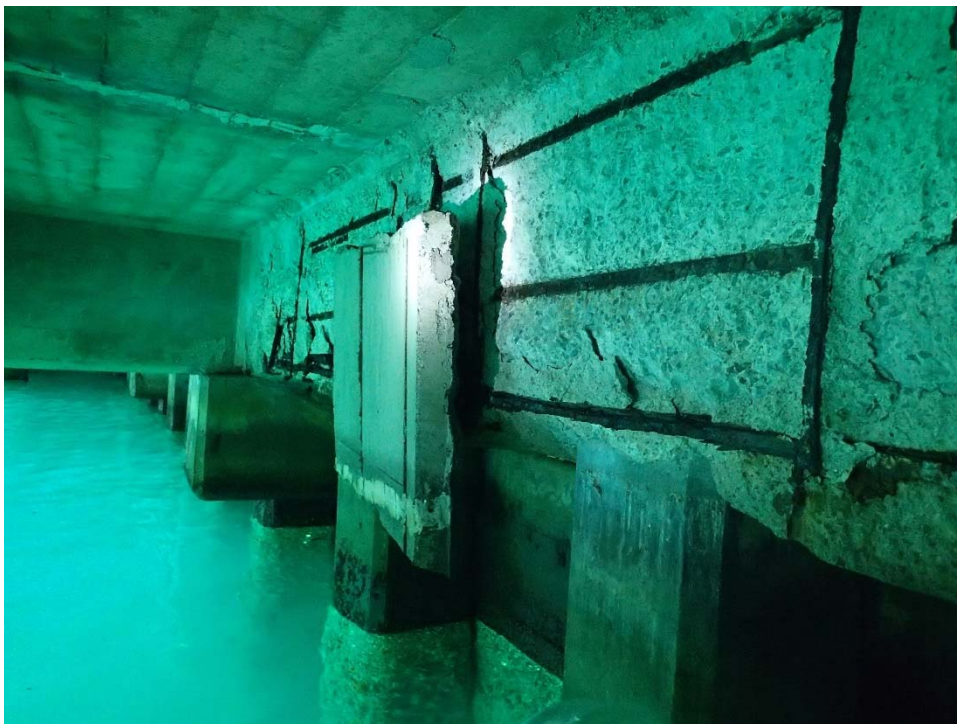
8 – Typical condition of the rear marginal beam with exposed and corroding reinforcing steel. The remaining portion of a previous beam repair area is shown hanging.
