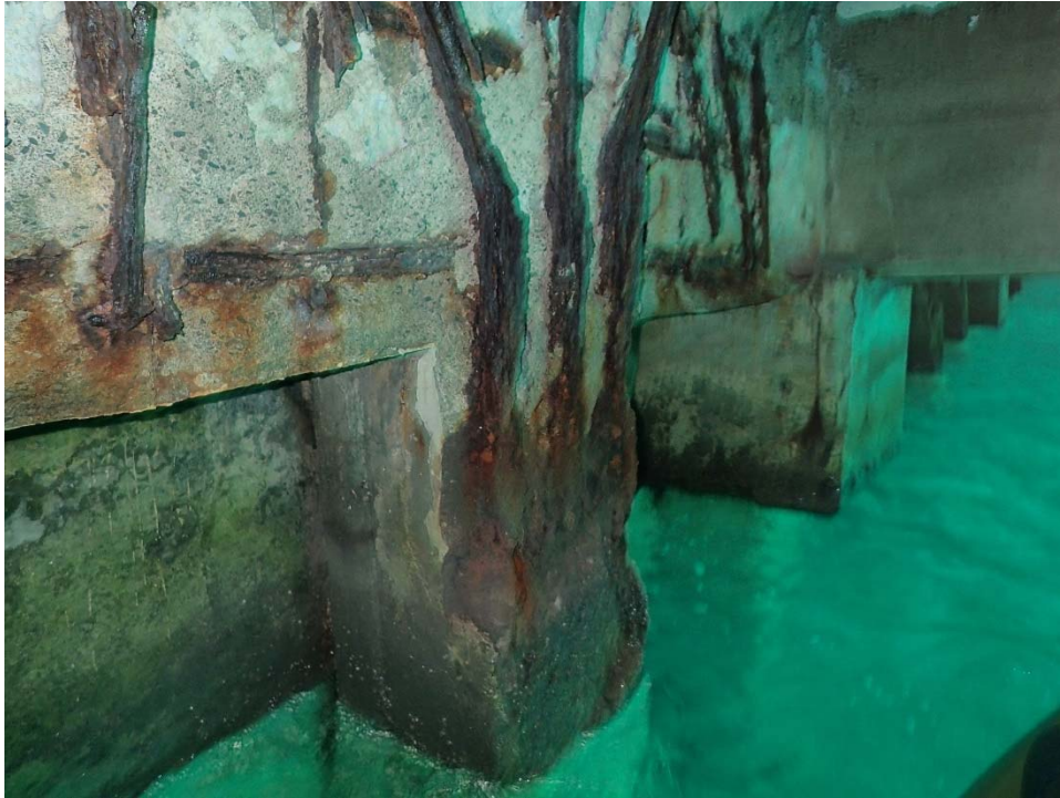
9 – Example of damage at the top of some piles along Gridline A (bulkhead) on the 1924 wharf.
