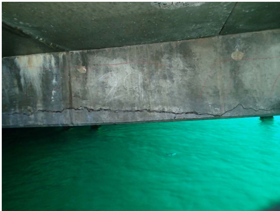
12 – Spalling along soffit of 1968 wharf pile cap
