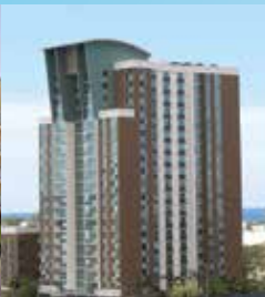
Halekauwila Place 665 Halekauwila 204 units, 204 R State Developed
