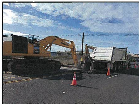
Paul's Electric doing trenching work connections between Langley and Monterey road.
