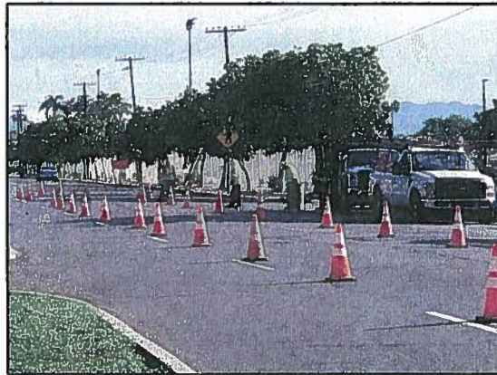
Paul's Electric begins duct work between Langley and Cord roads
