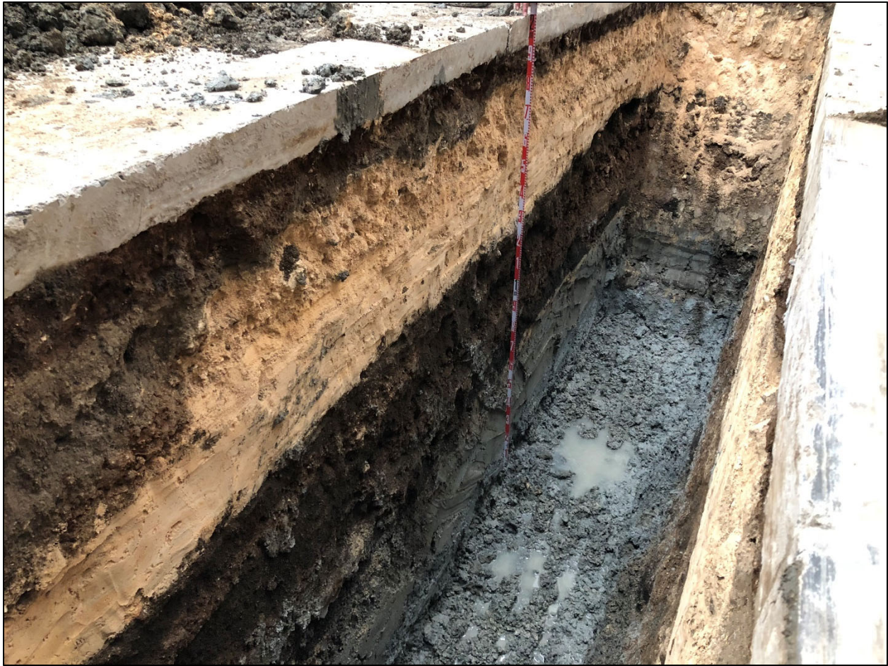
Figure 45. Photograph of T-6, west wall, view to southwest
