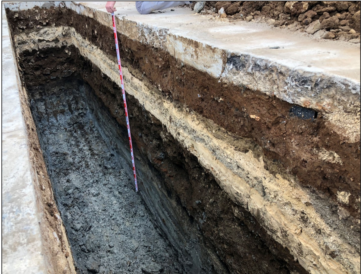
Figure 47. Photograph of T-7, southeast wall, view to east
