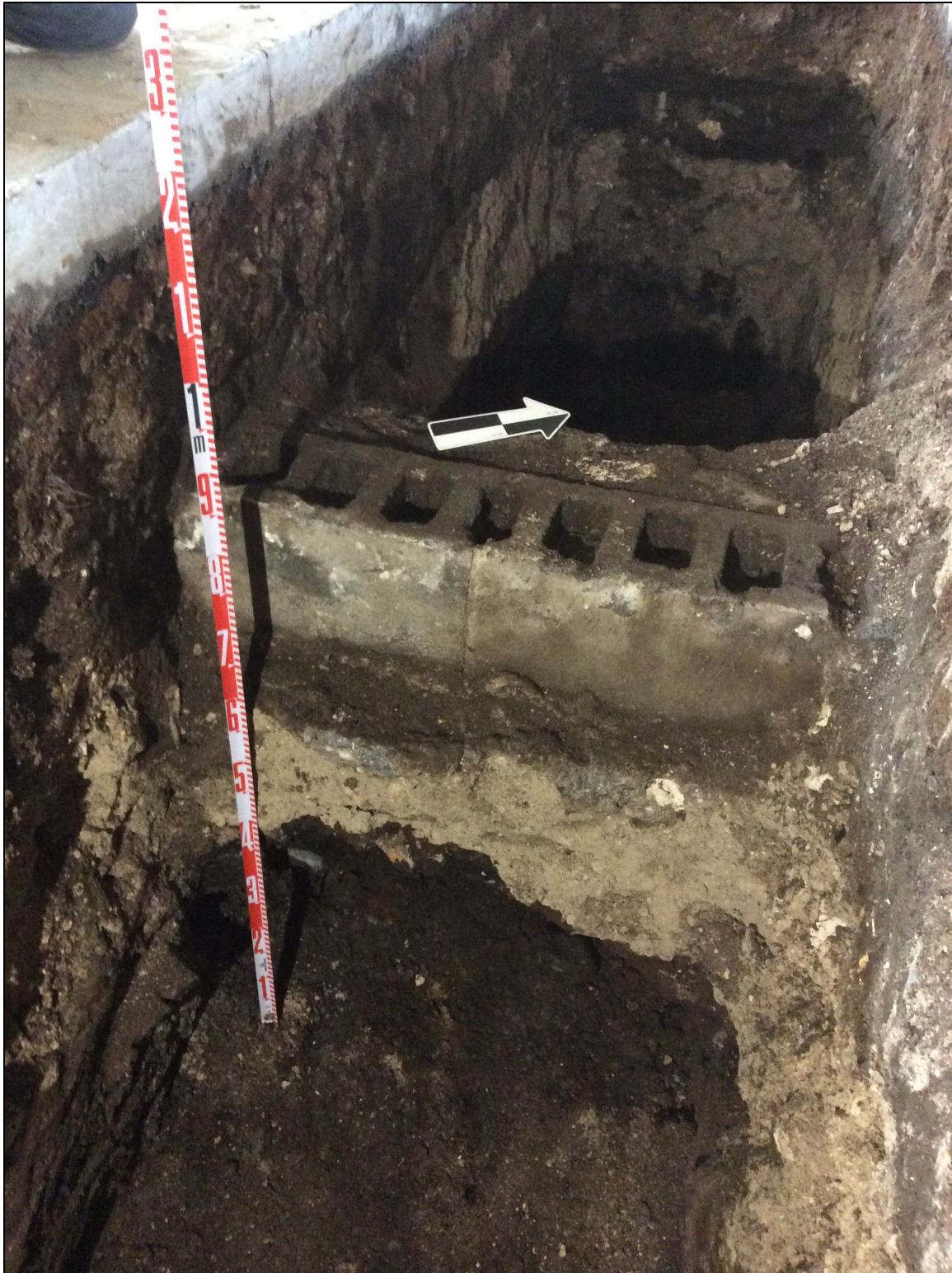
Figure B4. Photograph of SIHP # -8787 Feature 1, hollow tile footing, view to northwest
