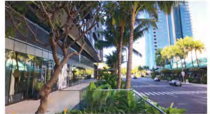
Kamake'e Street view corridor, as realized.
