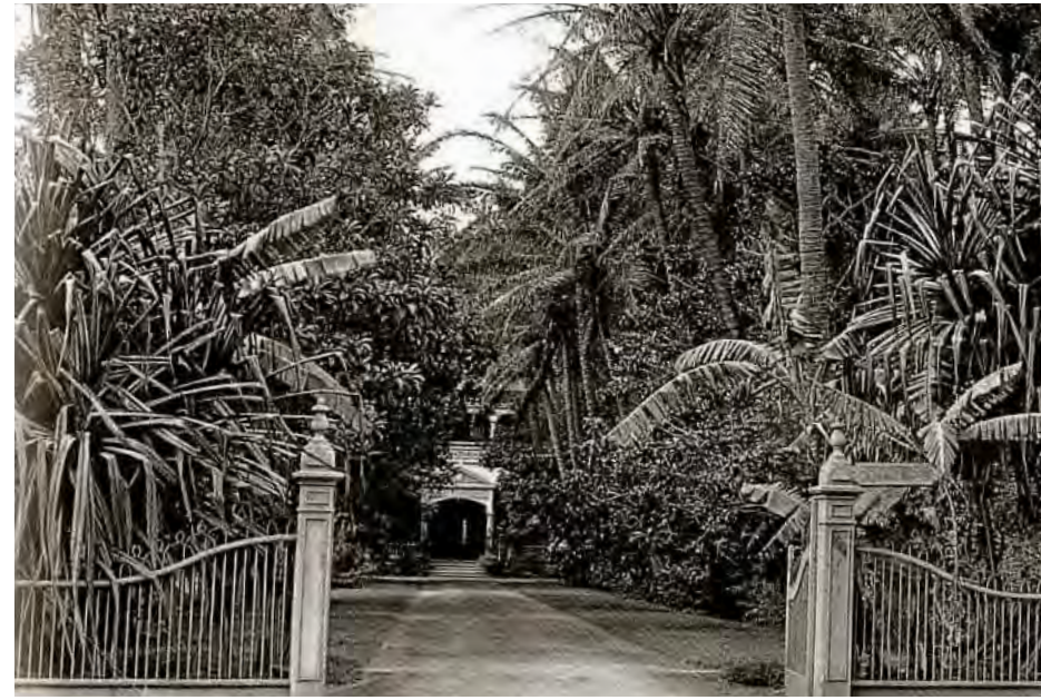
Victoria Ward's "Old Plantation" entrance, 1916.
