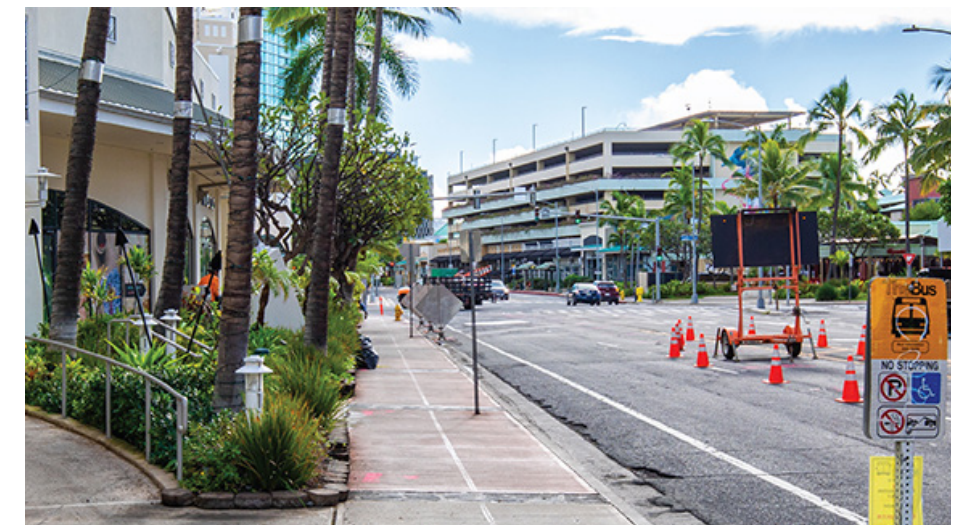
Current view of Auahi Street fronting Ward Entertainment Center.
