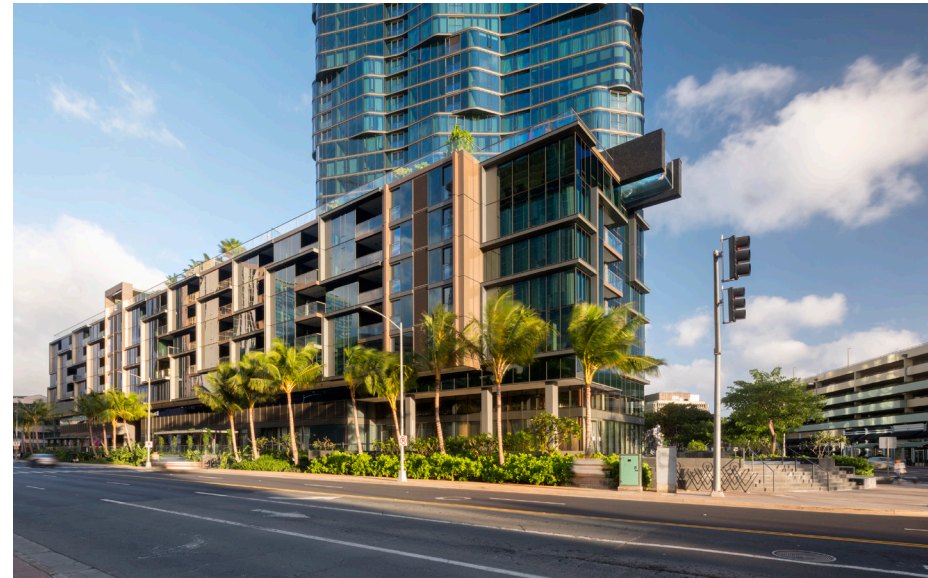
Ground floor restaurant and retail spaces of Anaha activate Kamake’e Street and Auahi Street.
