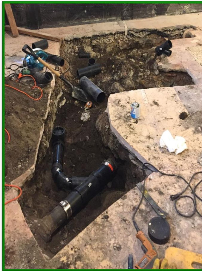
Figure 29: Example of Waste Piping
