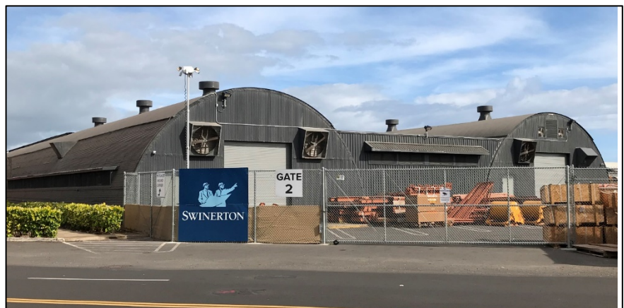
2021 photo by MASON showing the chain-link fence added along Enterprise Avenue, ca. 2019. Front façade modified with a larger opening for taller roll-up door.
