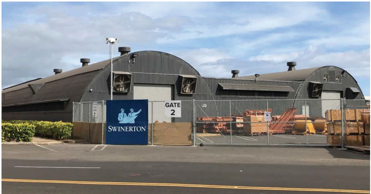
Fig. 4. View of existing fencing along Enterprise Avenue facade.
