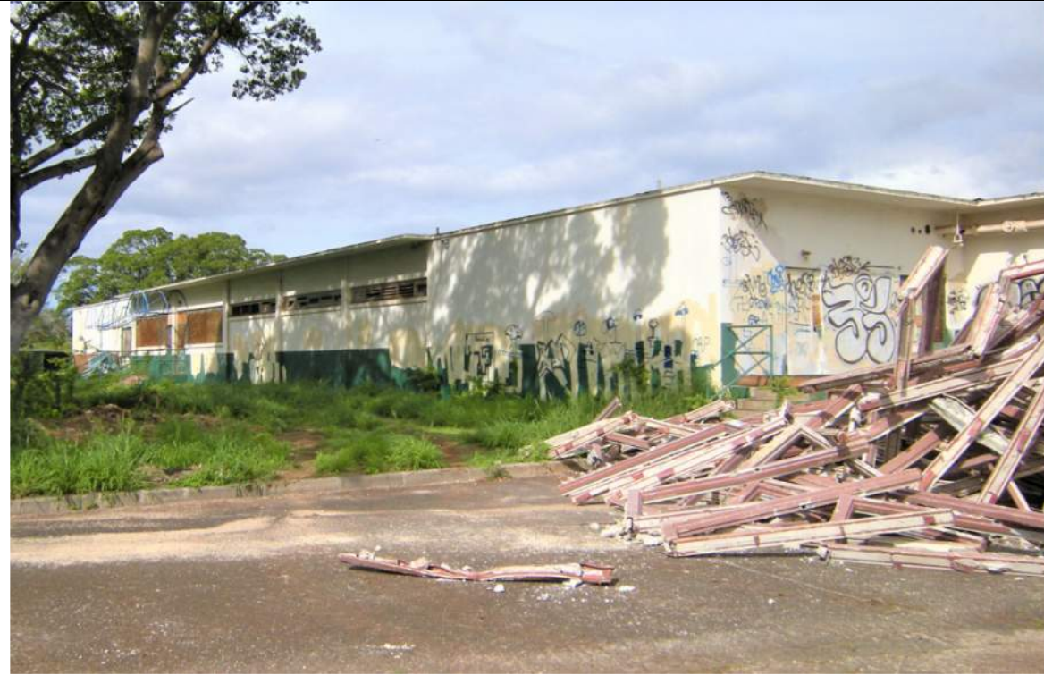
Fig. 7. (2014 Appearance.) Southeast corner.
