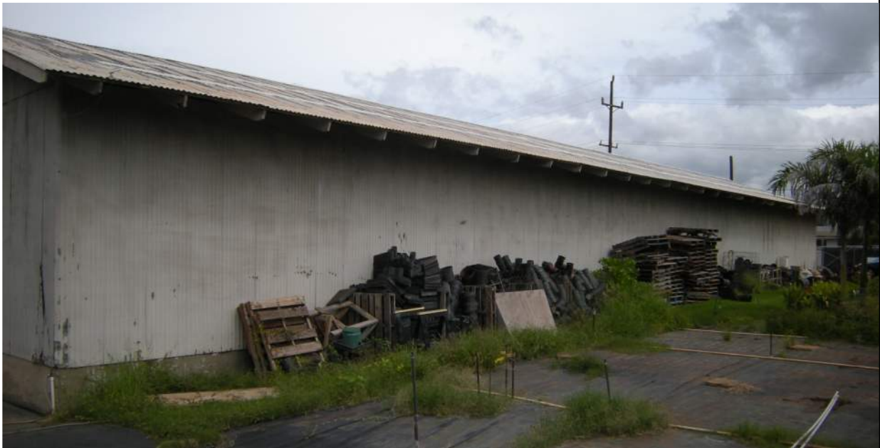
Fig. 3. Building 476, appearance of south side in 2014, with corrugated siding.
