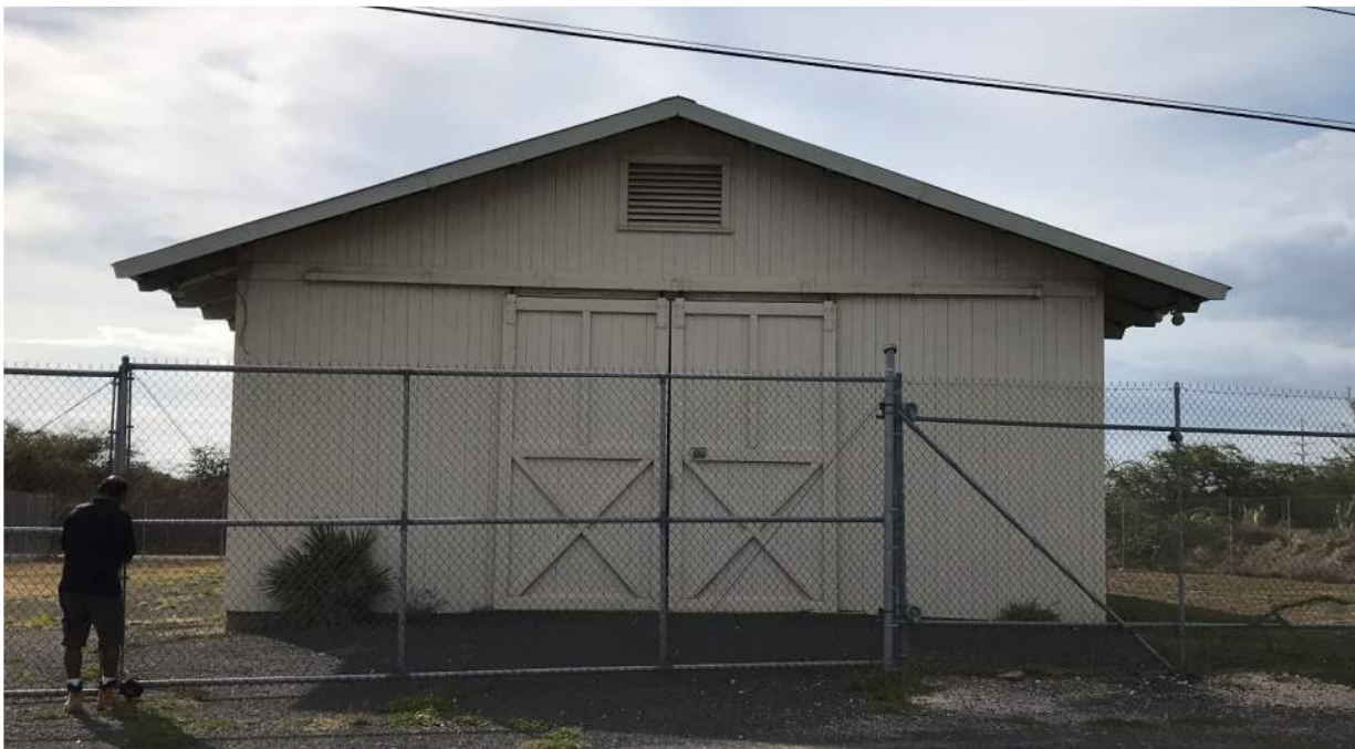
Fig. 8. Building 477, 2021 appearance. Historically appropriate repairs were made by the Navy in 2017.
