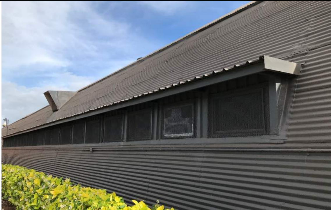
Fig. 8. (2021 Appearance.) View of character-defining window today (unchanged).
