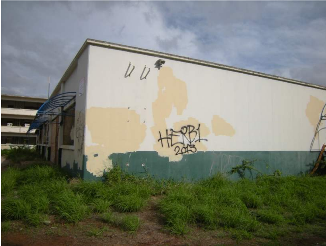
Fig. 3. (2014 Appearance.) Southwest corner.
