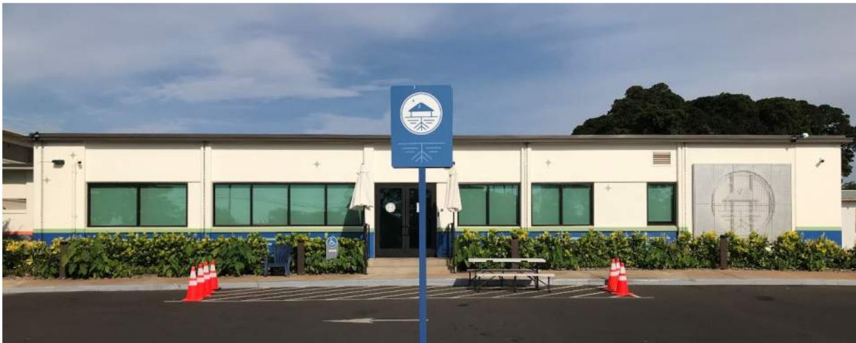
Fig. 2. (2021 Appearance.) The five-bay façade has been altered. The frames of historically inappropriate shade awnings were removed. The building entrance was moved into the center bay of the façade. The former entrance bay was partly infilled with a fixed panel as well as 3 windows, and the original steps were removed. The southernmost-bay was completely infilled; all windows were removed. The new central entrance is smaller than original, has a new stair with an aluminum rail with glazing. New windows with inappropriate blue/green tinting were installed.
