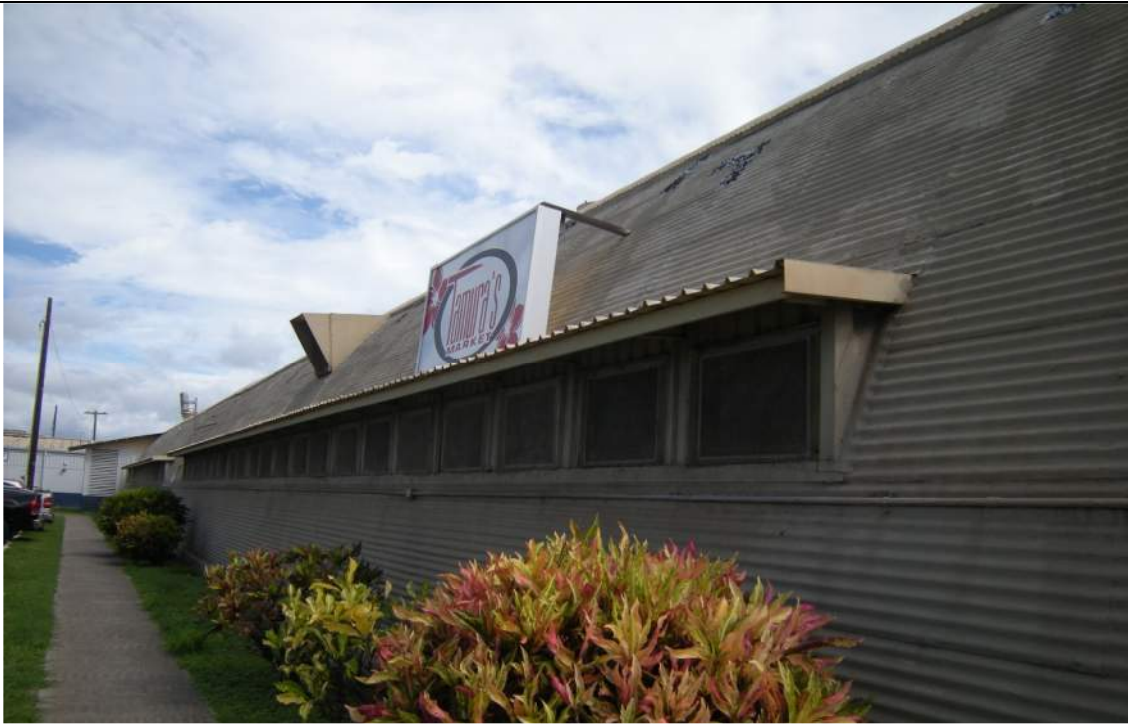
Fig. 7. (2014 Appearance.) View of character-defining window row, 2014.
