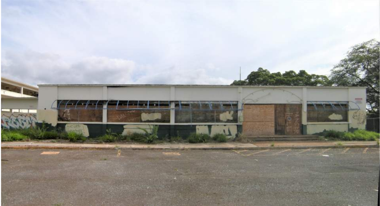
Fig. 1. (2014 Appearance.) When MASON last surveyed this building, it was abandoned. Windows and doors were boarded up, materials had been stripped, and it was covered in graffiti. Remnant frames of historically inappropriate shade awnings were attached above select doors and windows.
