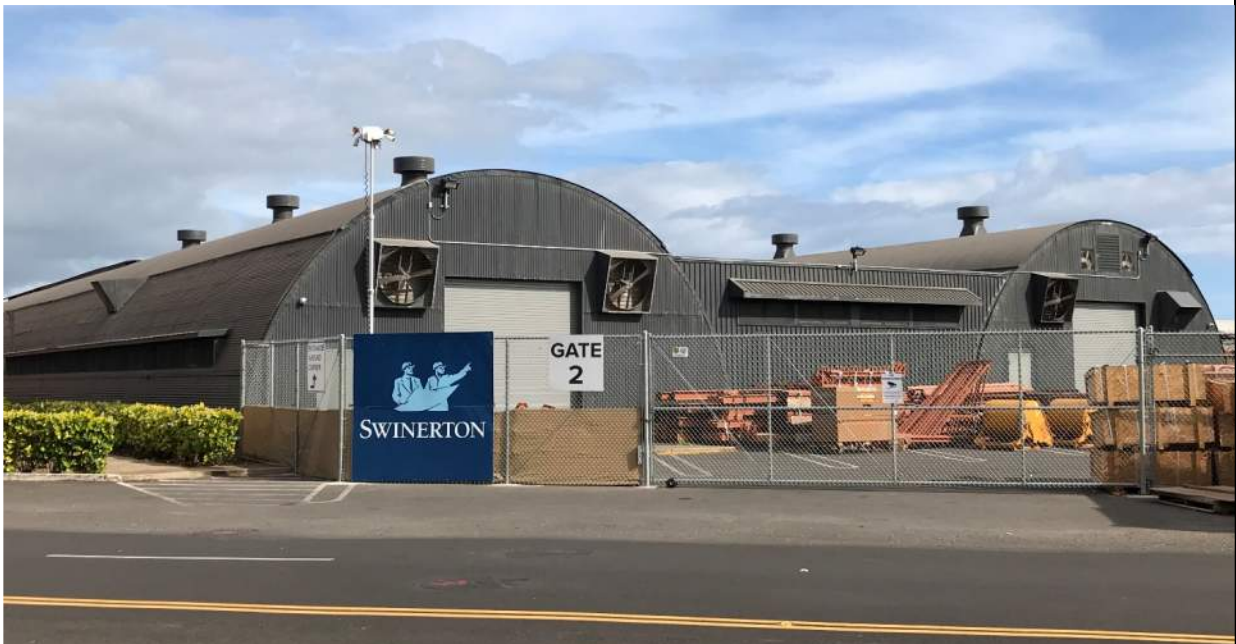
Fig. 2. (2021 Appearance.) View of Enterprise Avenue façade in 2021. Note the large-scale door at left is now the same height as the door on the right, and a fenced enclosure has been added under Phase 1.
