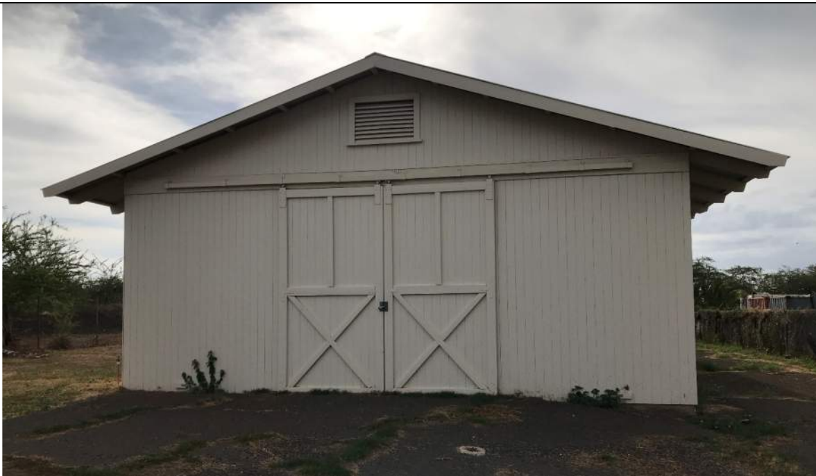
Fig. 2. Building 476, 2021 façade (view from Nassau Street). Hunt undertook building repairs in 2019 in an historically appropriate manner. The corrugated siding was replaced with wood siding. While a different material, the wood boards are historically appropriate, since both corrugated metal and wood were used as siding material in the dispersed storage buildings built at NASBP during World War II. The corrugated metal roof was replaced in-kind. Large-scale doors were reconstructed in an historically appropriate manner.
