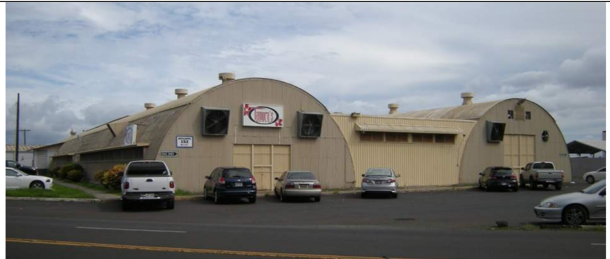
Fig. 1. (2014 Appearance.) View of Enterprise Avenue façade in 2014. Note the large-scale door at left is shorter than the door on the right and had been that way since at least 1965. (See Fig. 9)
