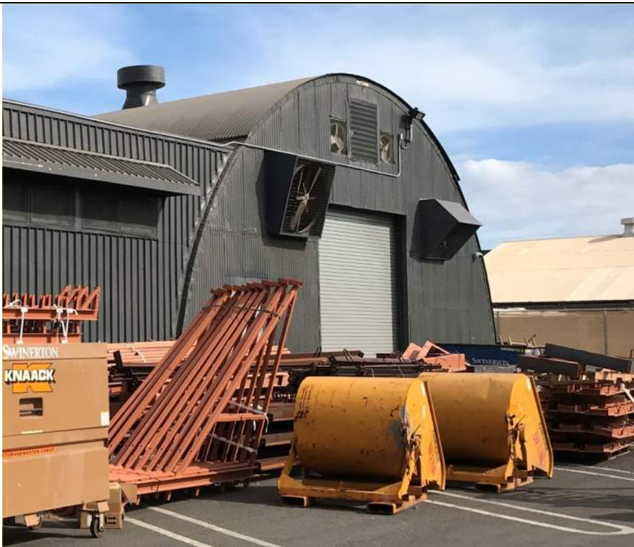
Fig. 6 (2021 Appearance) View of Enterprise Avenue façade in 2021 showing fenced enclosure and the replacement (roll-up) door, which is taller in height than the historic period door. (Phase 1)
