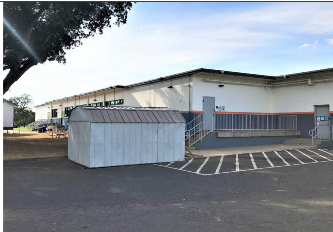
Fig. 7. (2014 Appearance.) Southeast corner. Original handrail was removed and replaced with new.
