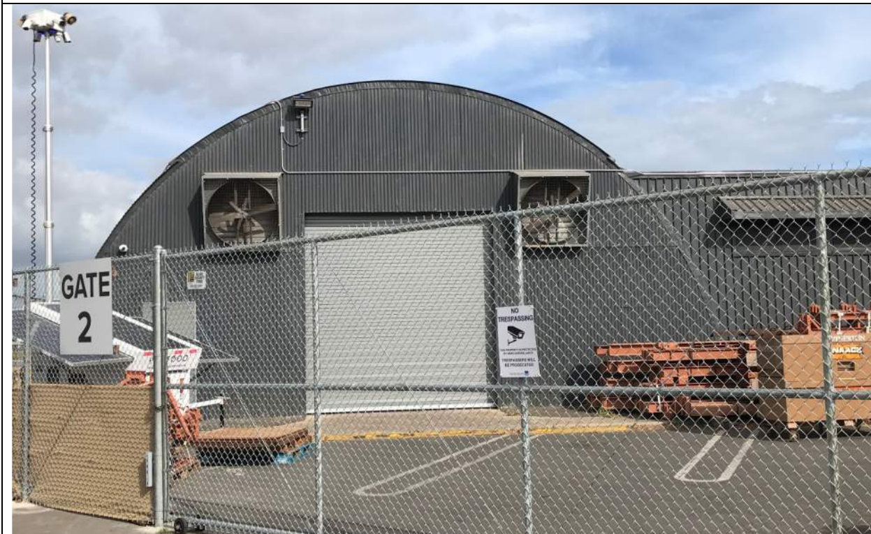
Fig. 4. (2021 Appearance.) View of Enterprise Avenue façade in 2021 showing fenced enclosure and the replacement (roll-up) door changes made in Phase 2. New door is taller in height than the historic period.
