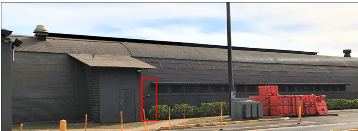
Proposed new door, overhang, and concrete stoop location marked with red box on 2021 photo by MASON.
