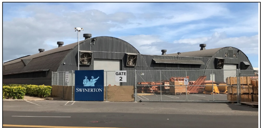
2021 photo by MASON showing the chain-link fence added along Enterprise Avenue, ca. 2019. Front façade modified with a larger opening for taller roll-up door.
