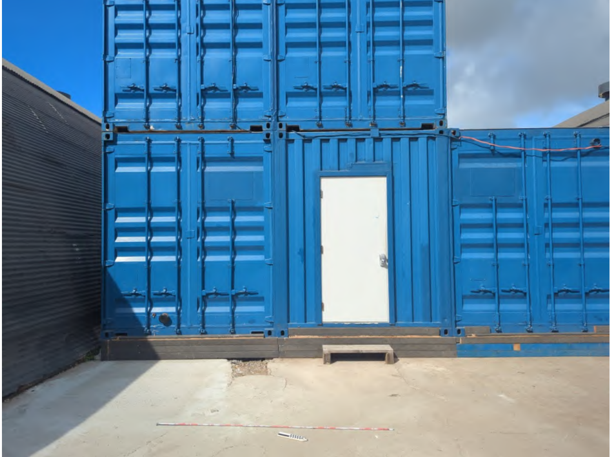
Photo 33 – Previous location of removed tank; view west-southwest
