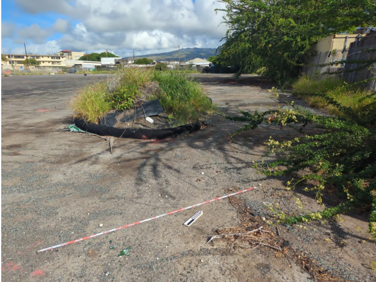
Photo 8 – View of asphalt parking lot, southeast corner of parcel; view north-northwest
