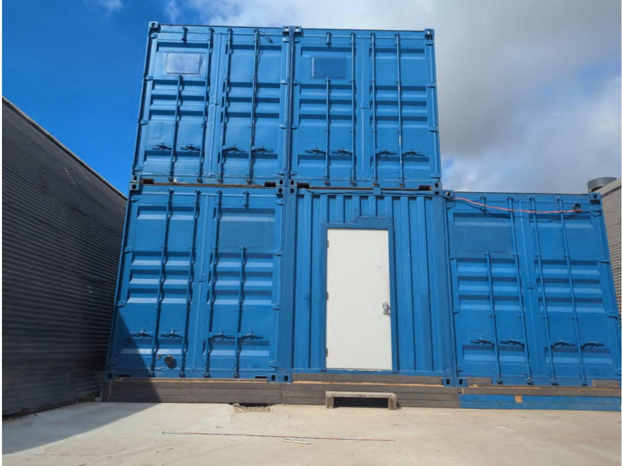
Photo 34 – Another view of previous location of removed tank; view west-southwest
