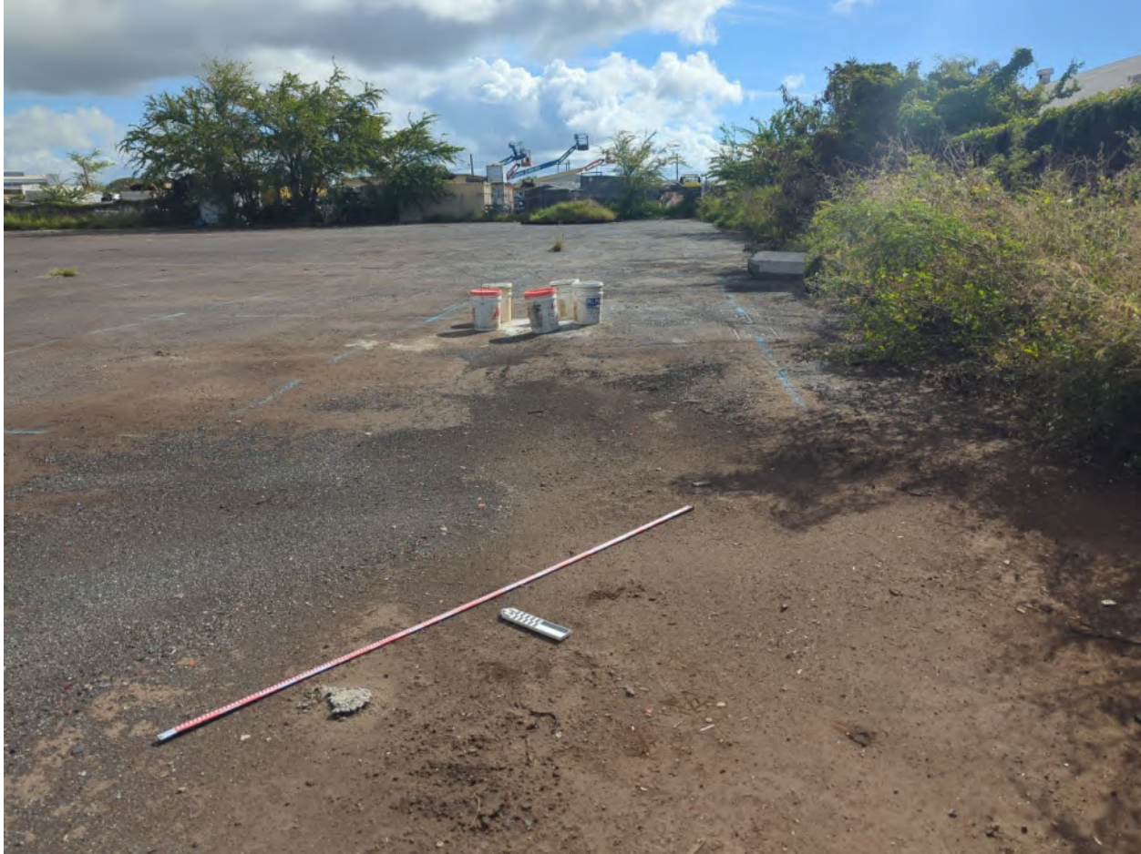
Photo 17 – View of southwest corner of asphalt parking lot in eastern portion of parcel; view northeast
