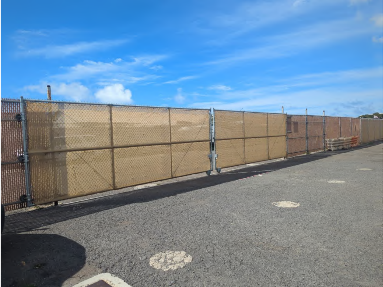
Photo 40 – Another view of southwest corner of parcel; view north
