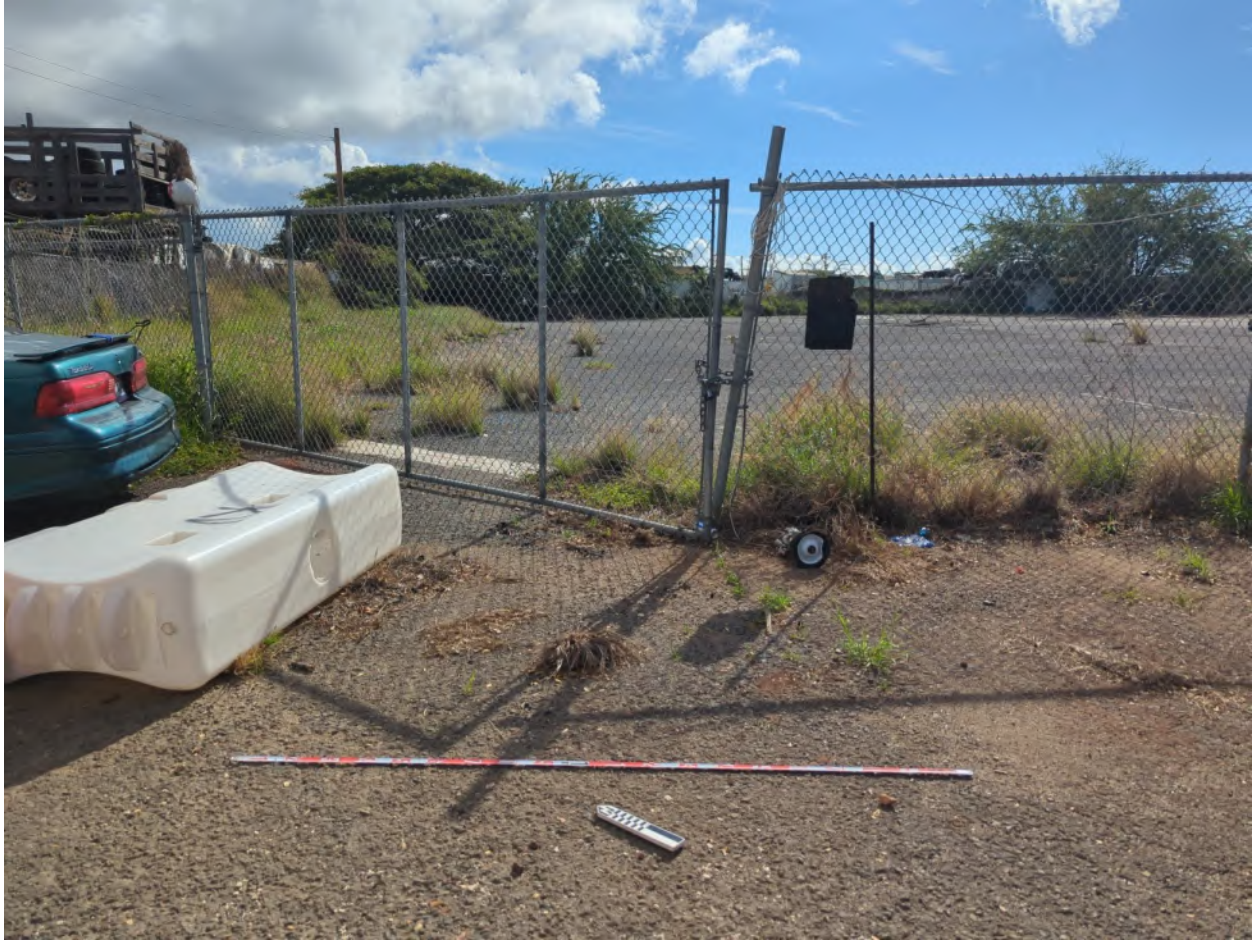
Photo 1 – Gated entrance to asphalt parking lot in eastern half of the parcel along Monterey Street (to the left); view northeast
