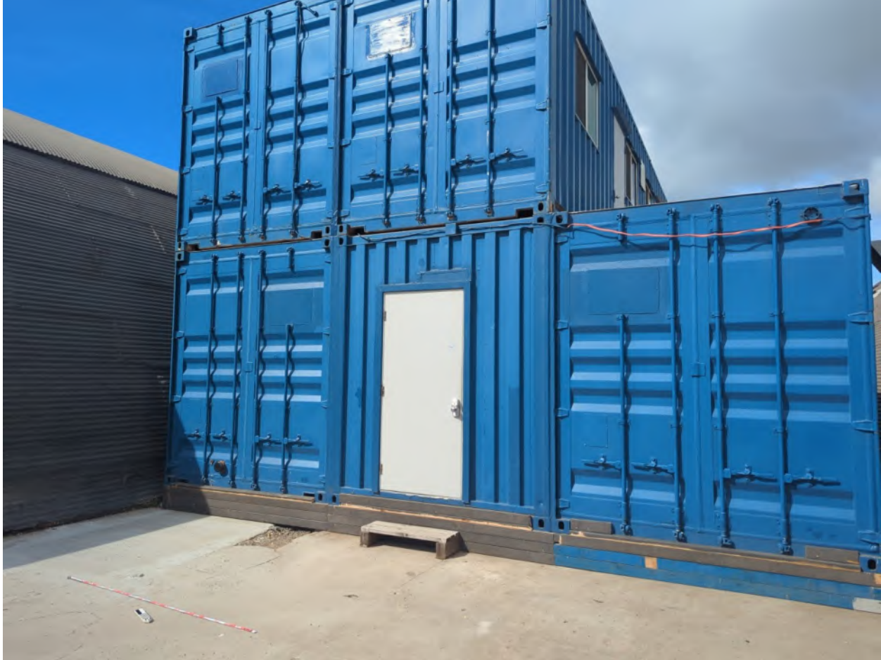
Photo 35 – Another view of previous location of removed tank; view southwest
