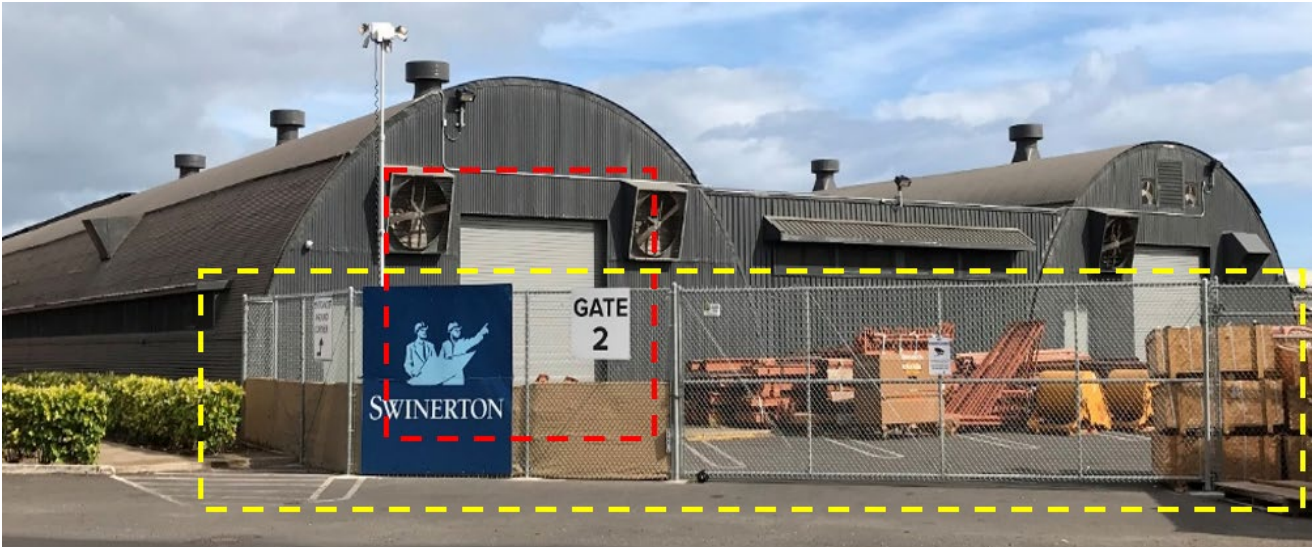
Figure 4 Photo of Facility 152 taken by MASON in 2021 with After-the-Fact work completed. The structure has been painted black. The enlarged exterior door is outlined in red and the new 8' fence is outlined in yellow.
