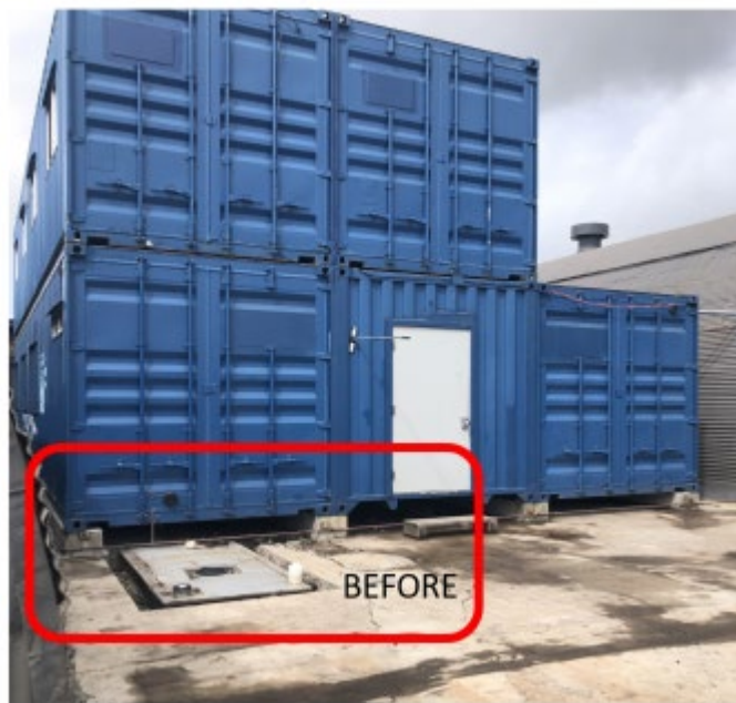
Figure 6 Swinerton (sublessee) installed a 250-gallon holding tank without HCH approval in 2021.
