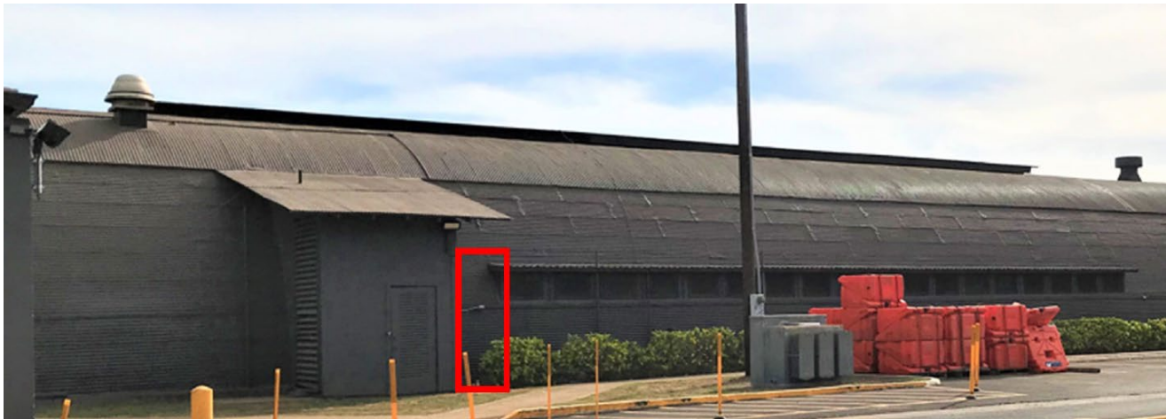
Figure 8 Proposed new door, overhang, and concrete stoop location outlined in red, on 2021 photo by MASON.
