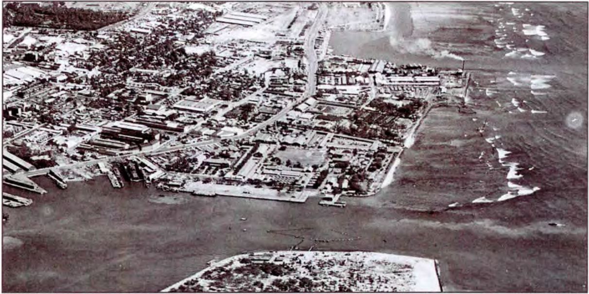
Figure 3: View of Kaka'ako Makai looking towards Diamond Head on October 31, 1942.
