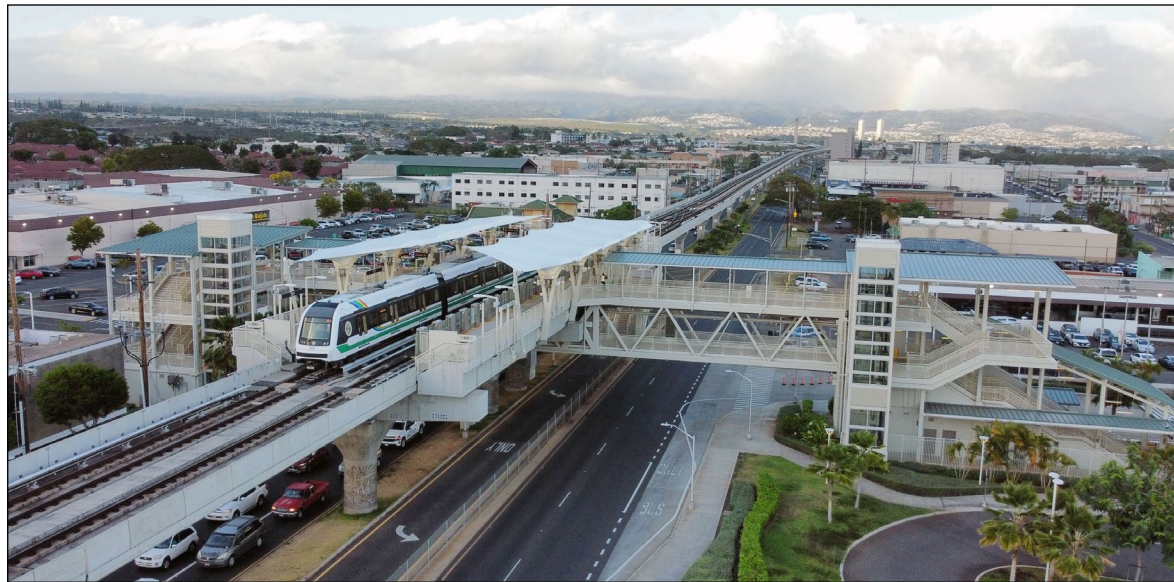
The Hō‘ae‘ae (West Loch) rail station serves as a mobility hub and is integrated into the urban fabric of Waipahu.
