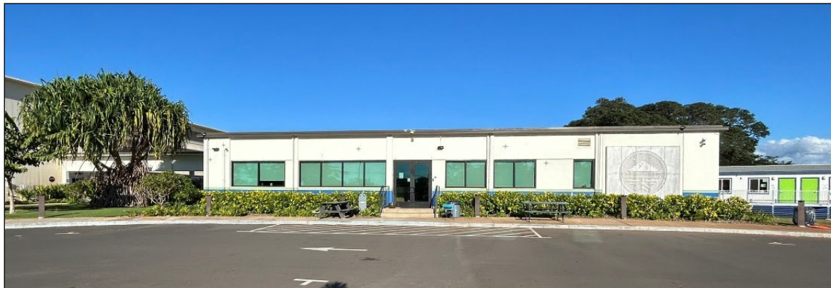
The DreamHouse Academy is located in rehabilitated former Bachelor Officer Quarters (BOQ) mess hall.
