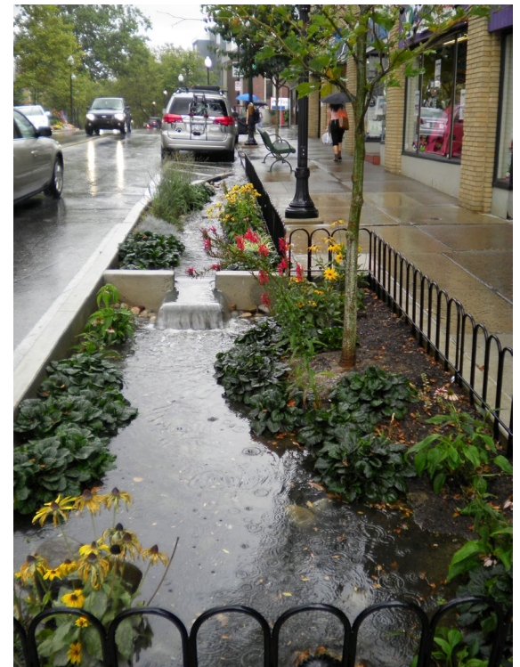
Rain gardens capture and treat stormwater while providing attractive landscaping in urban settings.
