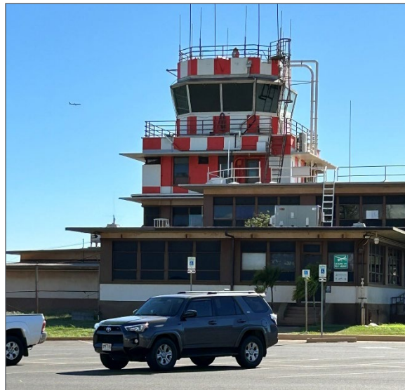
Kalaeloa airport control tower
