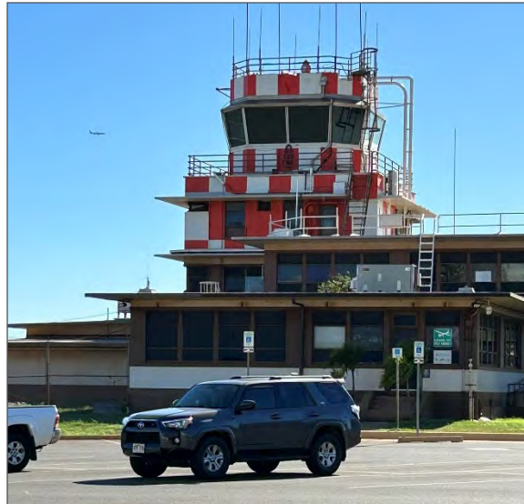
Kalaeloa airport control tower
