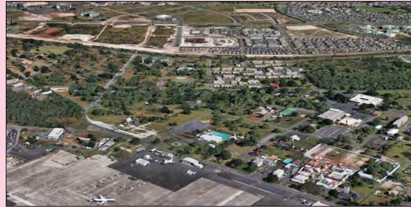
Figure 3-5: Existing conditions - mauka view
