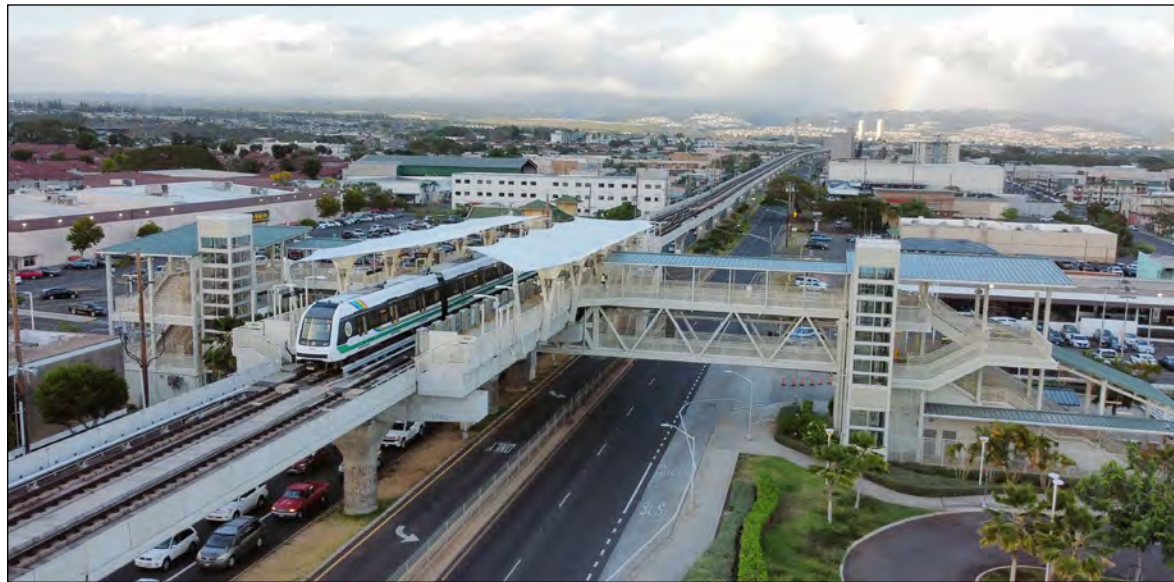
The Hō‘ae‘ae (West Loch) rail station serves as a mobility hub and is integrated into the urban fabric of Waipahu.
