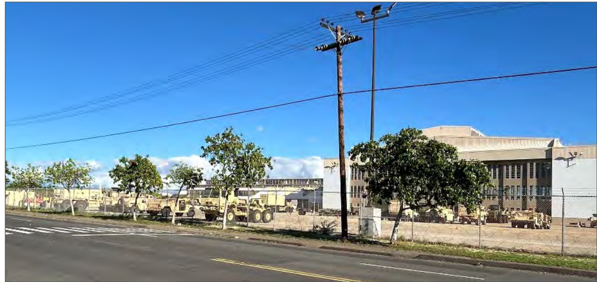
Street trees fronting Hawaii National Guard facility along Enterprise Street.
