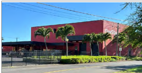
The former NEX furniture store was renovated for use as a transport and distribution business.
