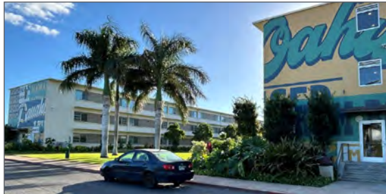
The Wakea Garden Apartments provides 100 units in the former Bachelor Officers Quarters (BOQ).
