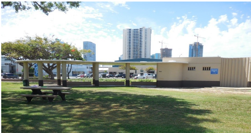
Figure 4.5: Comparative views of the comfort station and mauka pergola in 1937 (top) and 2016 (bottom). Note the modified block openings in the restroom wall and the two-color paint scheme.
