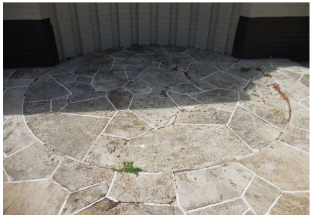
Figure 3.9 (top left): Flagstone paving beneath the pergola on the Halekauwila Street side of the comfort station. Figure 3.10 (top right): Flagstone paving for access to storeroom door. Figure 3.11 (left): Looking toward Pohukaina Street at the curved band of flagstone paving that connects the pergola walkways. Figure 3.12 (right): Distinctive circular paving joint on top of the circular platform at the center of the comfort station.
