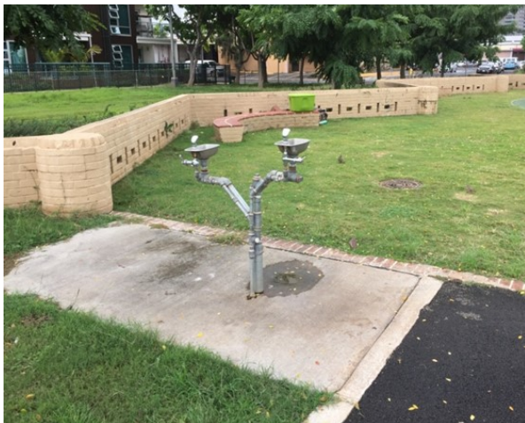
Figure 3.36 (top): Small scale features include the drinking fountain mounted on a poured concrete pad.
