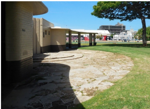
Figure 3.9 (top left): Flagstone paving beneath the pergola on the Halekauwila Street side of the comfort station. Figure 3.10 (top right): Flagstone paving for access to storeroom door. Figure 3.11 (left): Looking toward Pohukaina Street at the curved band of flagstone paving that connects the pergola walkways. Figure 3.12 (right): Distinctive circular paving joint on top of the circular platform at the center of the comfort station.
