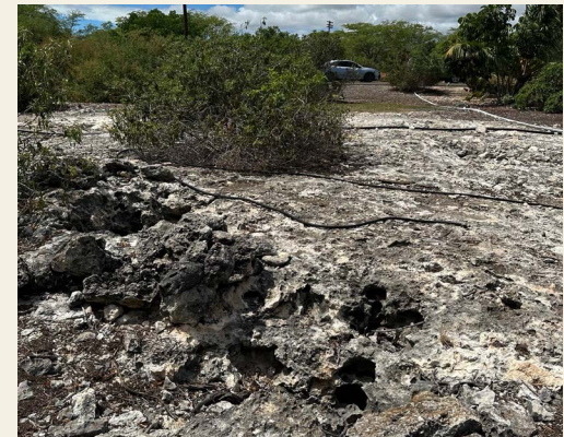
Remnants of a karst sinkhole
