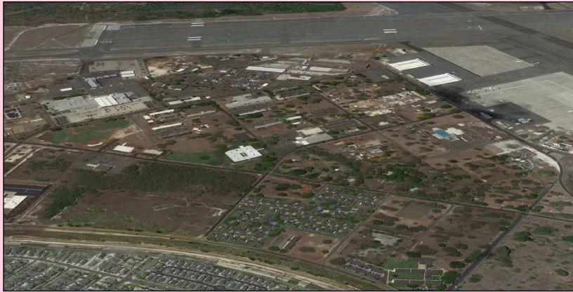
Figure 3-3: Existing conditions - makai view
