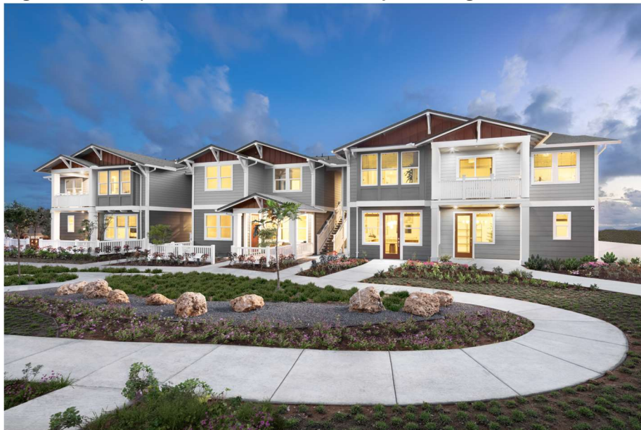
Figure B: Completed Ka‘ulu Multi-Family Building
