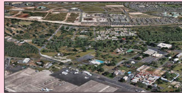
Figure 3-5: Existing conditions - mauka view
