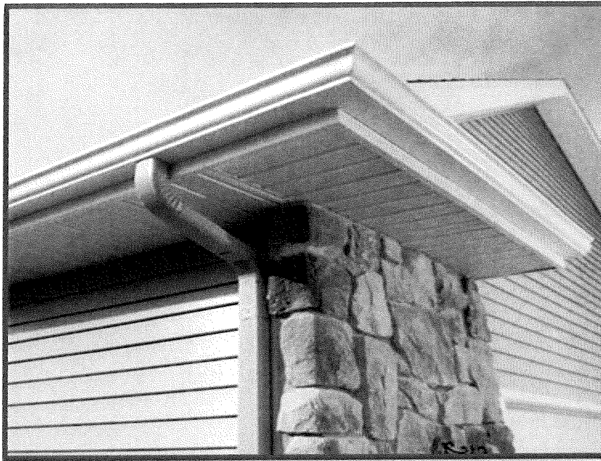
Figure 8: Example of Residential Gutter
