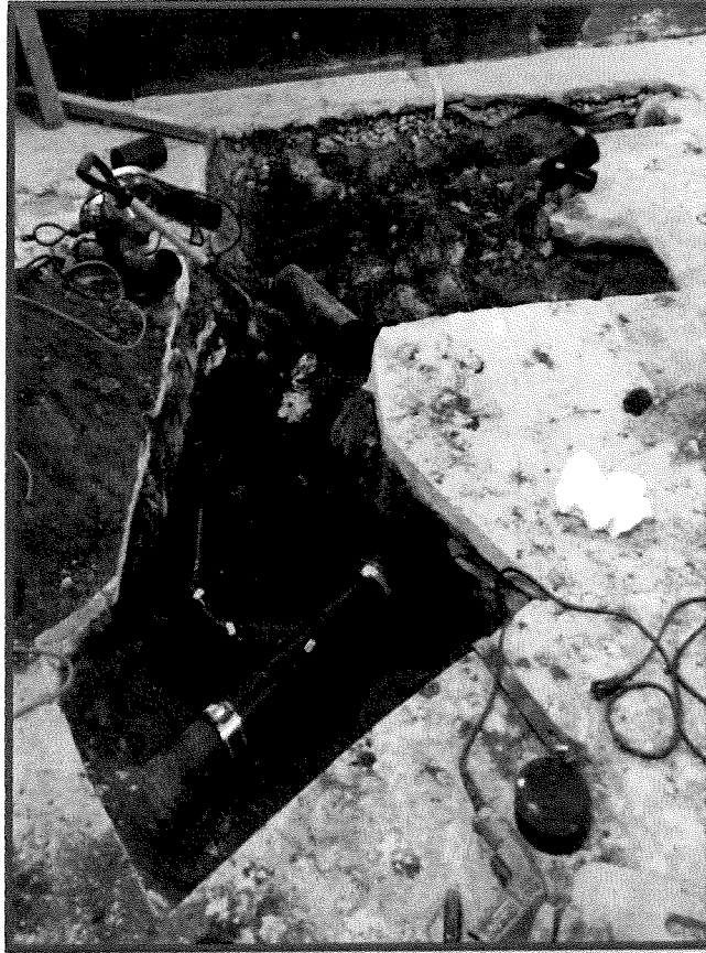
Figure 29: Example of Waste Piping
