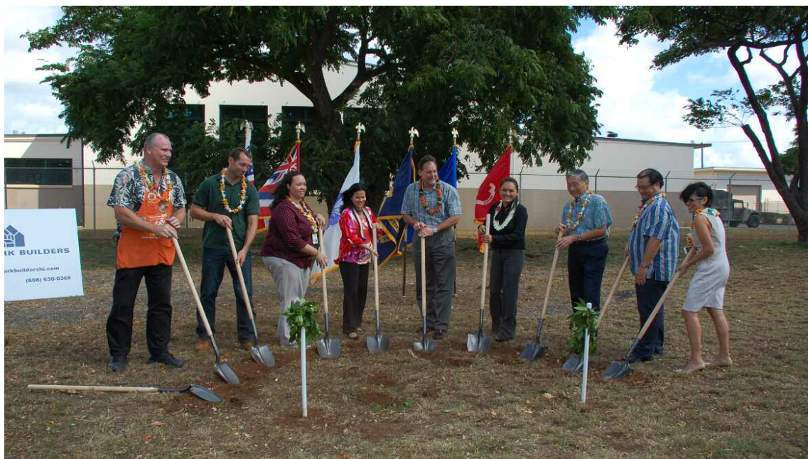
Hale Uhiwai Nalu Addition Groundbreaking for the 50-unit addition to Hale Uhiwai Nalu in Kapolei
