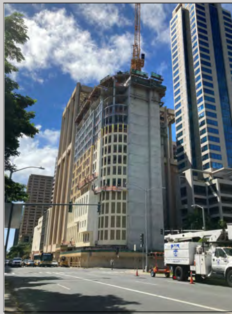
Kokua under construction, September 2022
